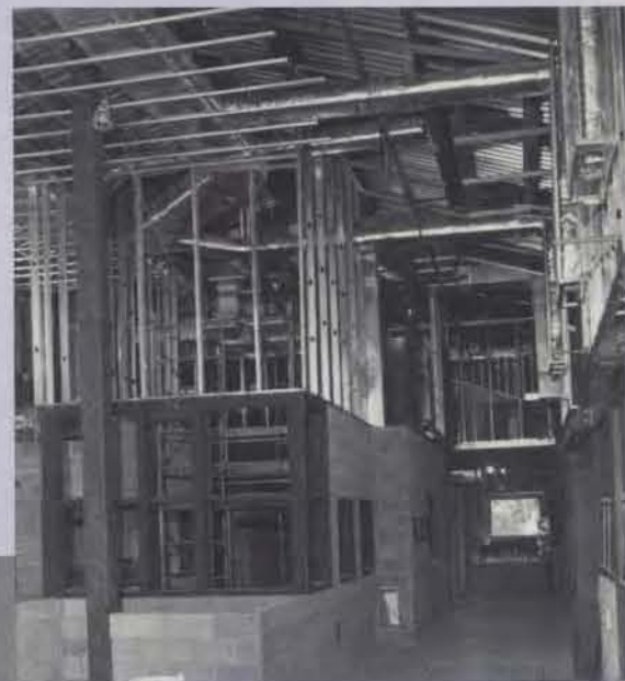
Interior of the building.
