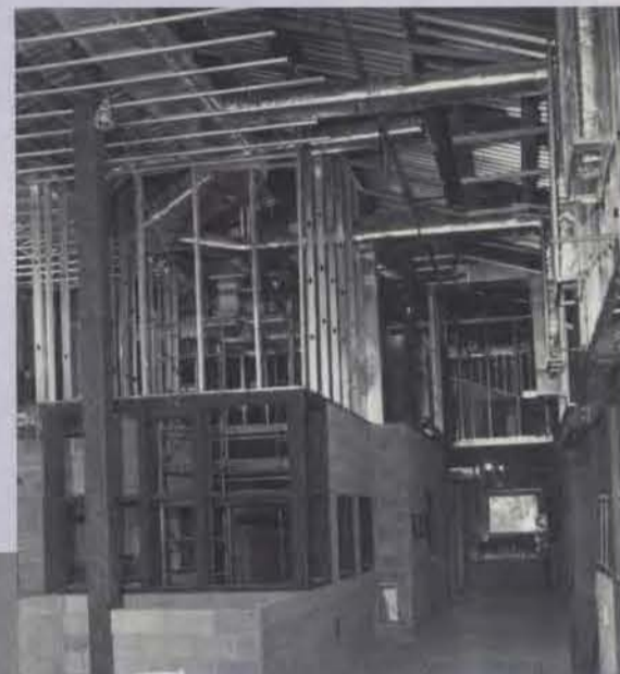
Interior of the building.
