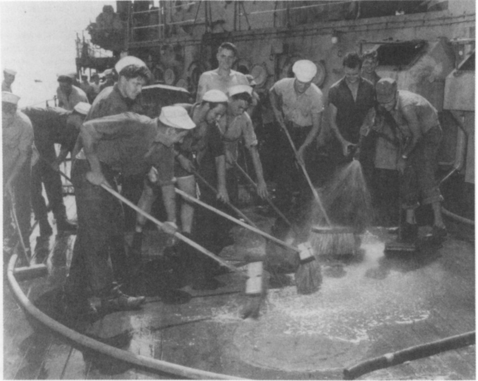
Sailors scrubbing the deck of the Prinz Eugen to reduce radiation levels after Operation Crossroads. The ship had been part of the "target fleet" in the 1946 atomic bomb test at Bikini Atoll (reprinted from Weisgall, Operation Crossroads).
