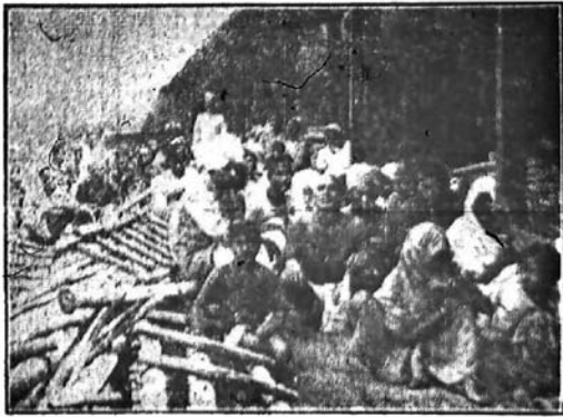
Refugees at the Mall Road Power House
