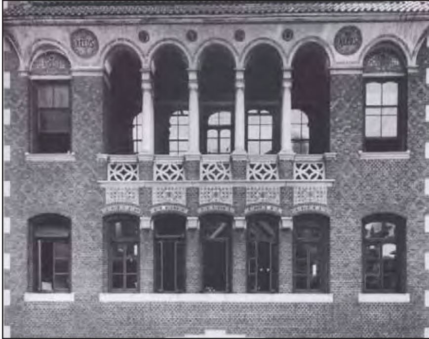
Image 3: Detail of Upper Loggia 1904
