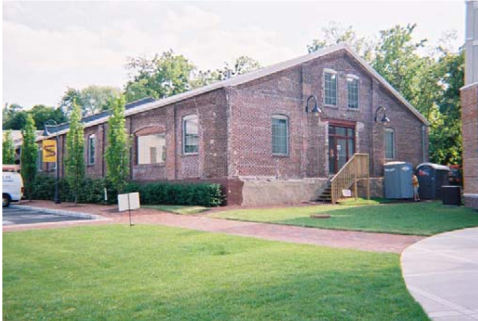
Figure 16-Union Square Development-Adaptive re-use project by George Michael Inc. preserved some older buildings but demolished most.
