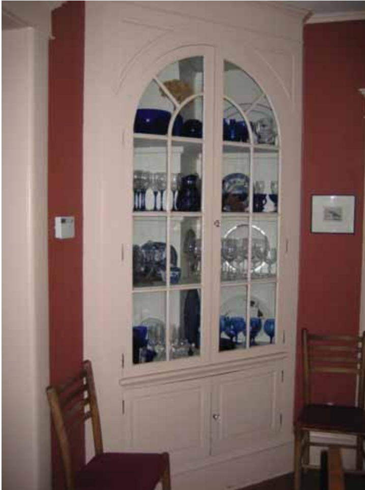
Figure 4.9: The existing dining room china cabinet, previously a fire place. (Author's photograph)
