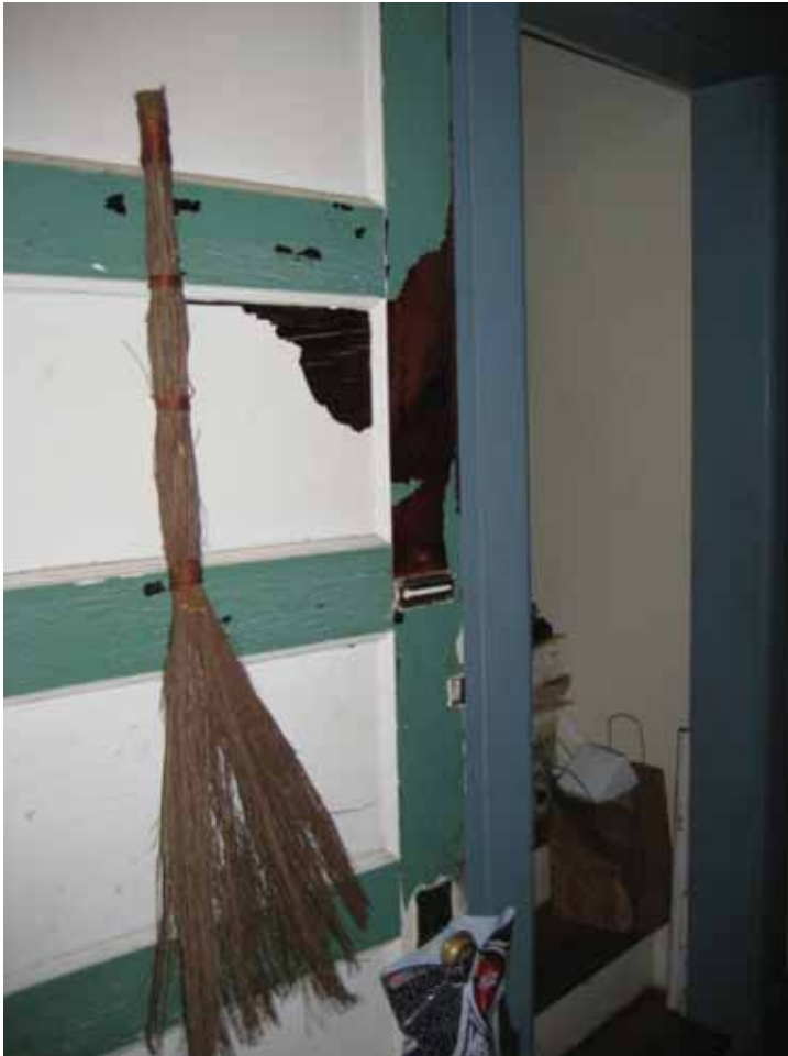
Figure 4.5: The door to the basement stair case (left) with the existing back stair case to the right. (Author's photograph)
