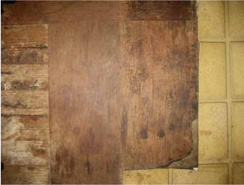
Figure 4.15: The flooring in the existing kitchen- possible original flooring (far left) with subflooring laid above (center of photo), and linoleum over the subflooring (far right). (Author's photograph)
