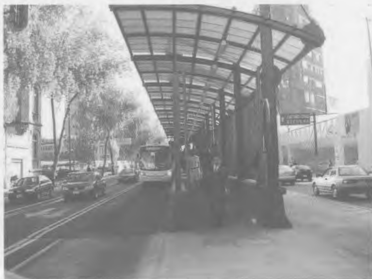
Fig. 12 The Bus Rapid Transit (BRT) in Mexico, a low-cost improvement attracted many passengers from cars and mini buses
