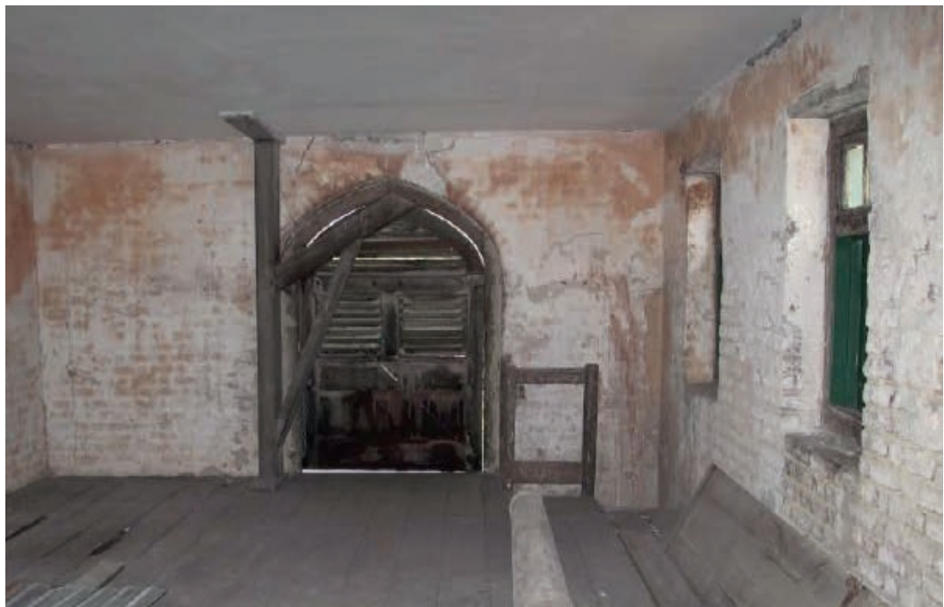
Figure E: Aiken-Rhett Stables: Second Floor North Chamber, with orange limewash still visible. 38
