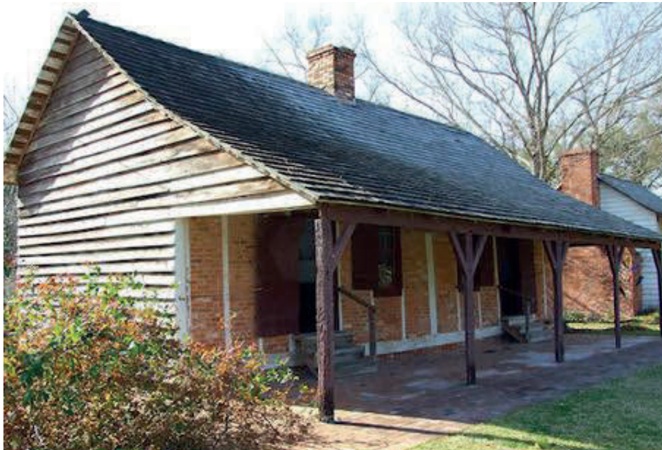
Figure T: Kent Plantation Slave cabin: brownish-red timbers lining porch 169
