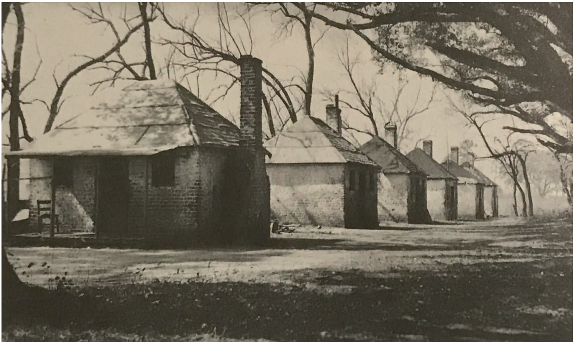
Figure Q: Brick slave cabins at Hermitage plantation, Georgia 110
