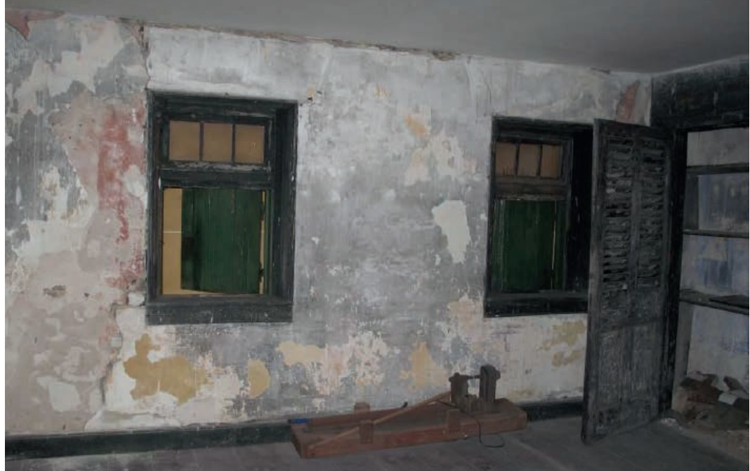
Figure C: Aiken-Rhett Stables: Second Floor South Chamber, louvered closet door. 36
