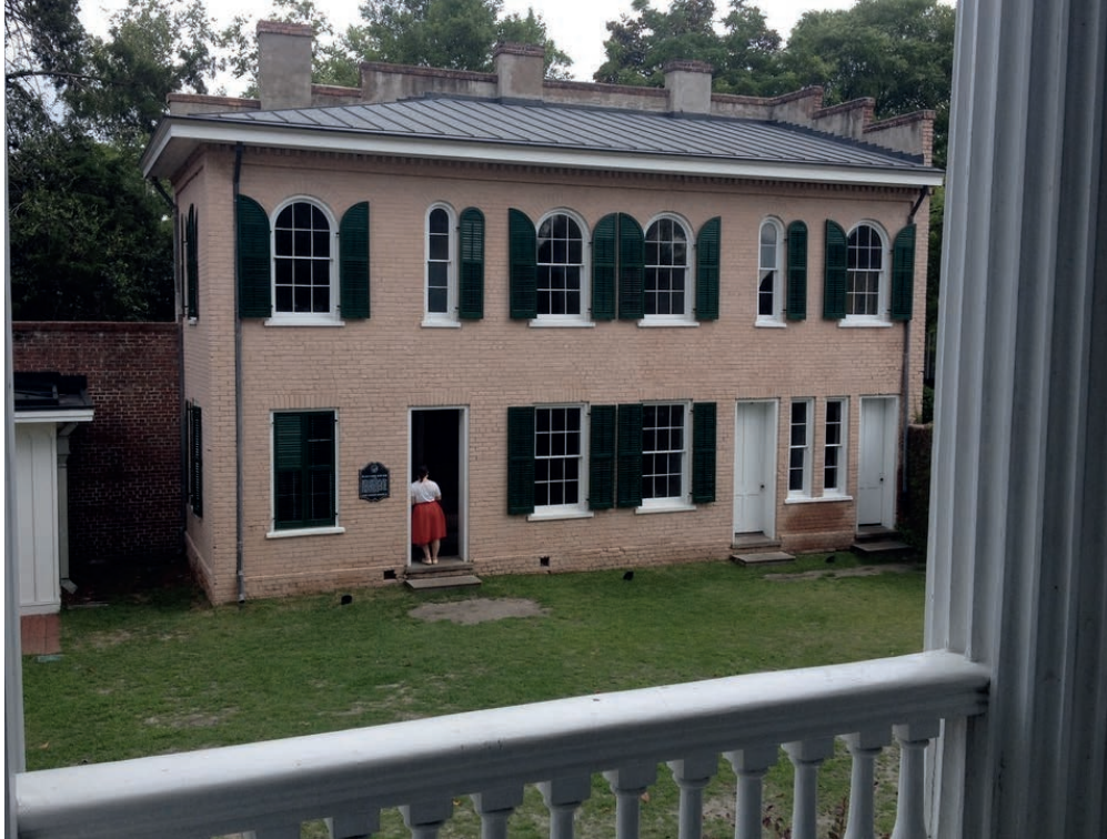
Figure K: Bellamy Mansion Slave House, restored: as seen from the back porch of the main house 58
