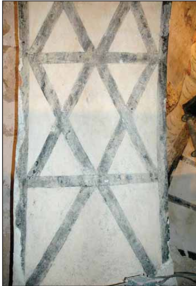
Figure 2.5: Black banding and intersecting cross pattern on intrados of arch (Source: Johnston and Silva, 14).
