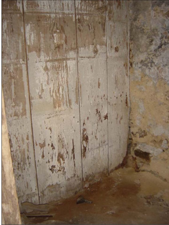
Figure 6: Ventilated closet in Northeast room depicting evidence of shelves (Higgins, 2006).
