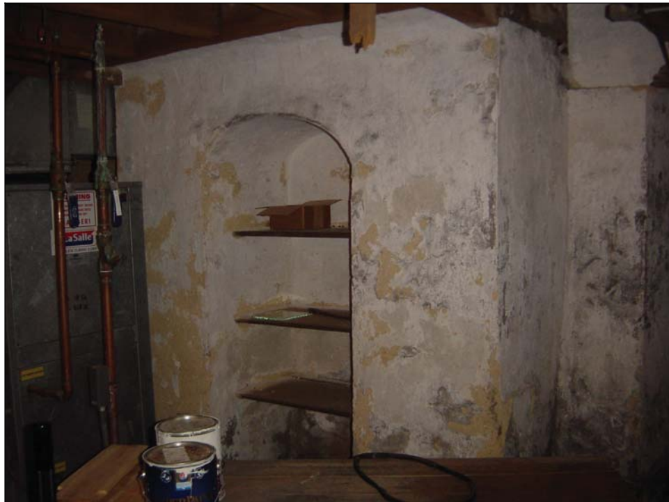
Figure 15: Arched storage recess in dairy (Higgins, 2006).
