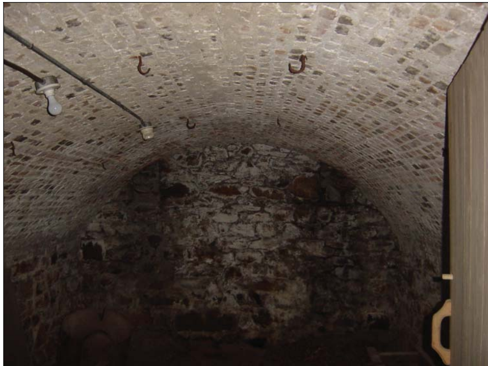
Figure 13: Wrought iron hooks in ceiling of Central South room (Higgins, 2006).
