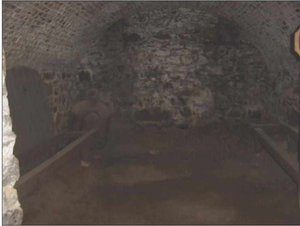
Figure 12: Central South room (Higgins, 2006).
