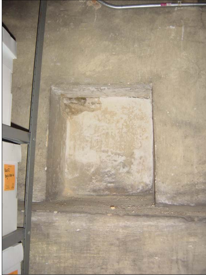
Figure 11: Niche 4 in Southeast room (Higgins, 2006).
