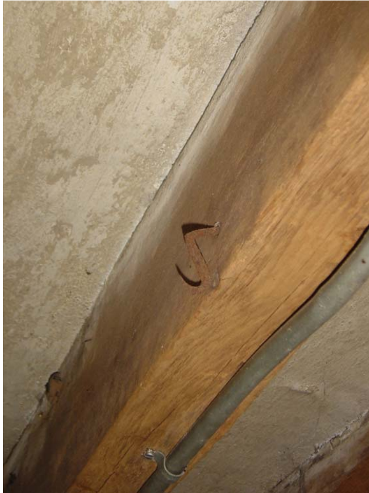
Figure 18: Wrought iron hooks in dairy (Higgins, 2006).
