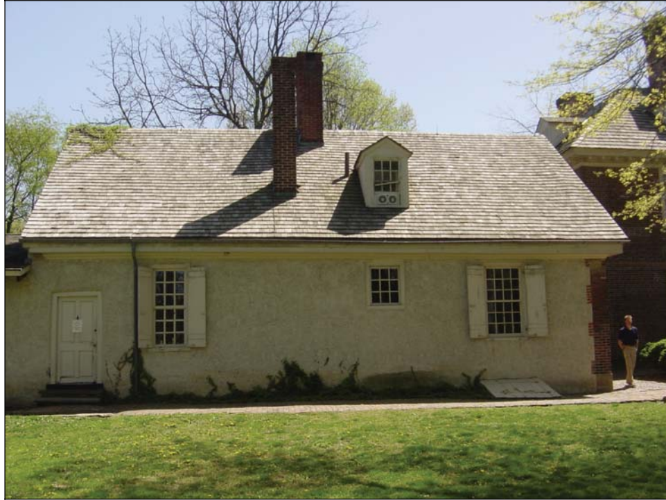
Figure 22: West elevation of the kitchen wing. The second floor housed the interior smoking room, between the two chimney stacks. (Higgins, 2006).
