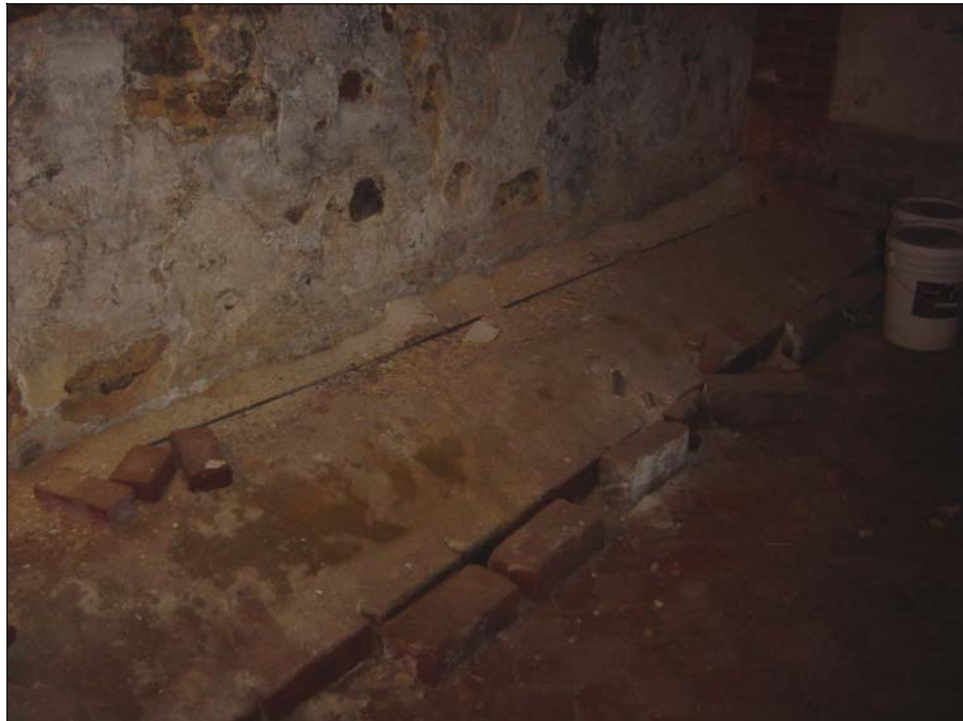
Figure 17: Trench along North wall in dairy (Higgins, 2006).
