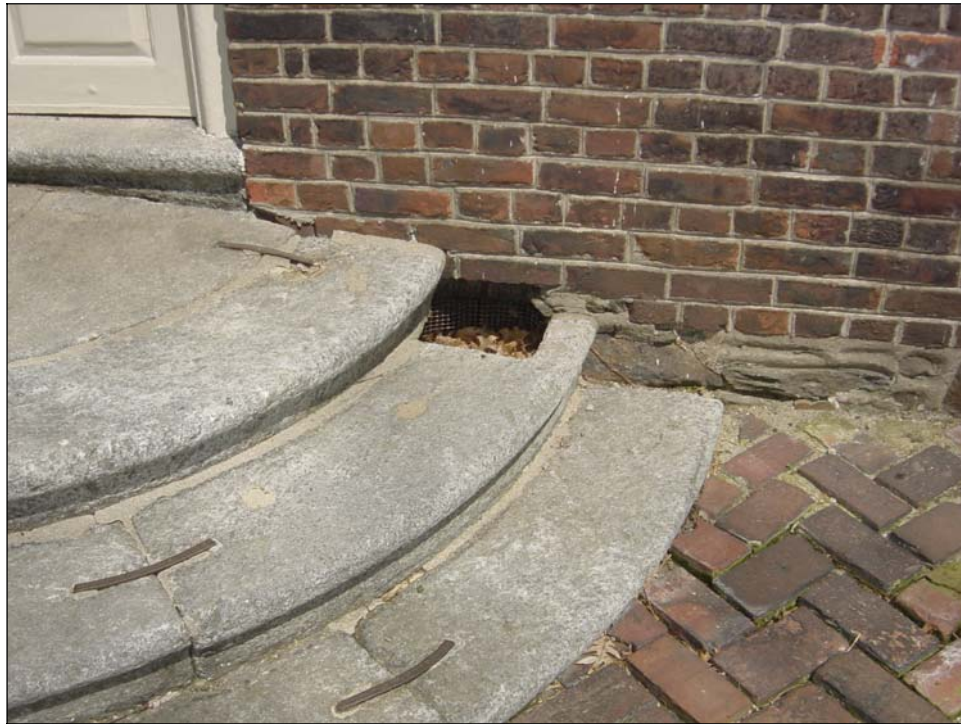
Figure 14: Ventilated windows to Central South room, exterior view (Higgins, 2005).
