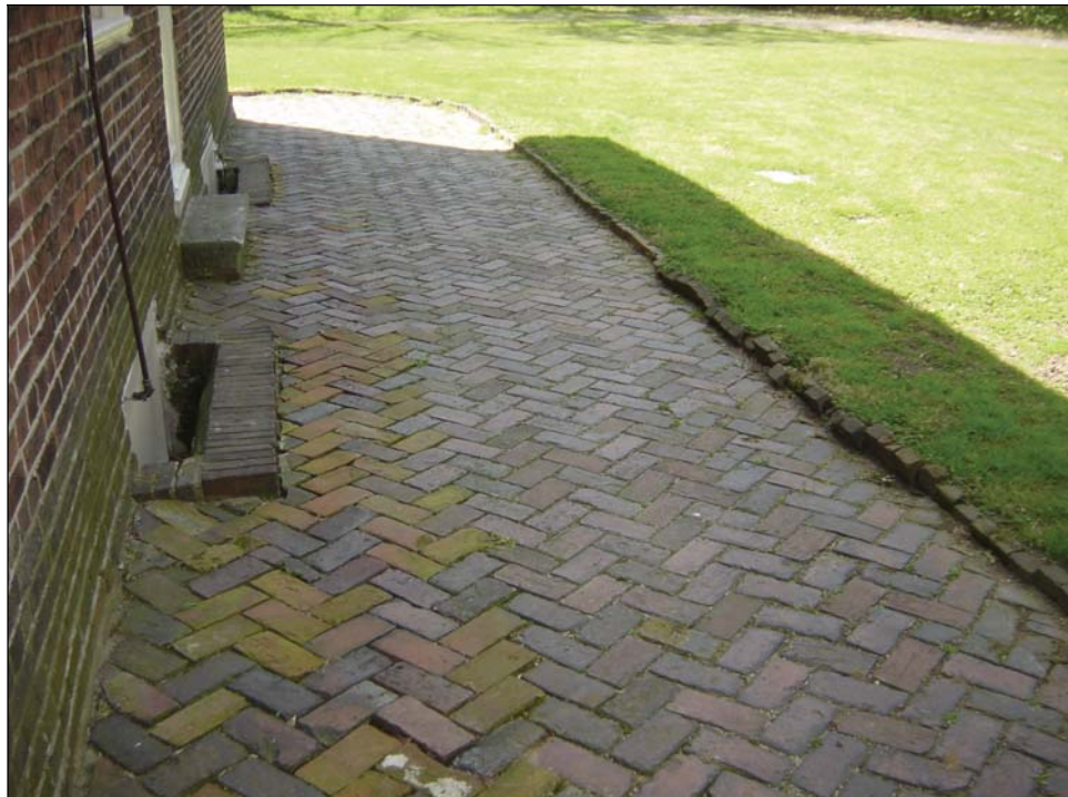
Figure 24: Exterior herringbone brick pattern. This same pattern is found in the foyer of the main house, and in the dairy, or Northwest room (Higgins, 2006).
