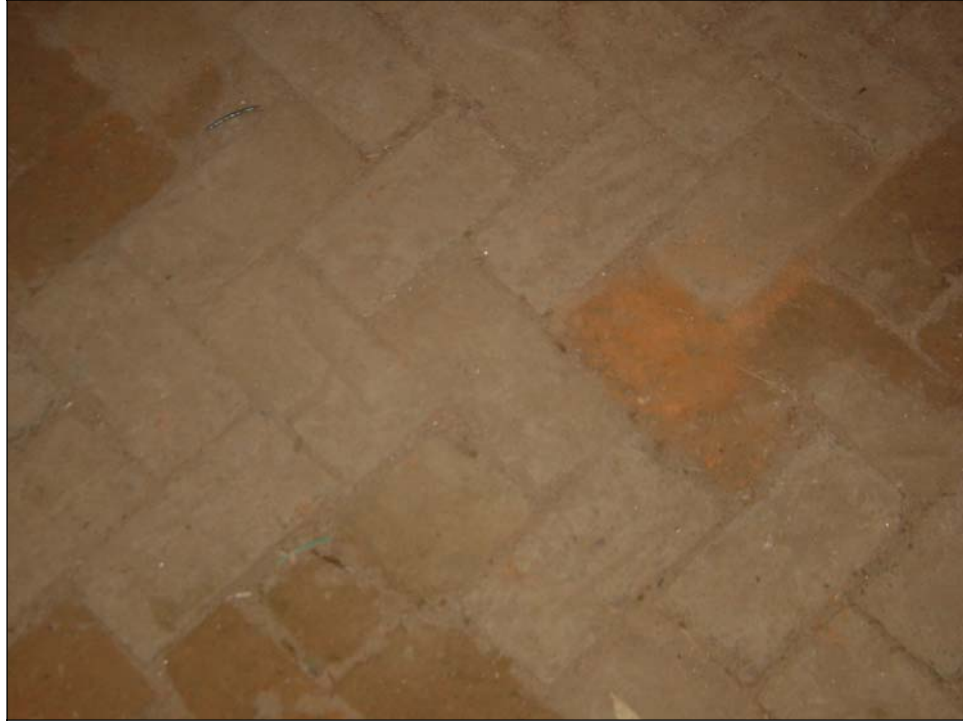
Figure 23: Herringbone patterned brick floor in dairy (Higgins, 2006)
