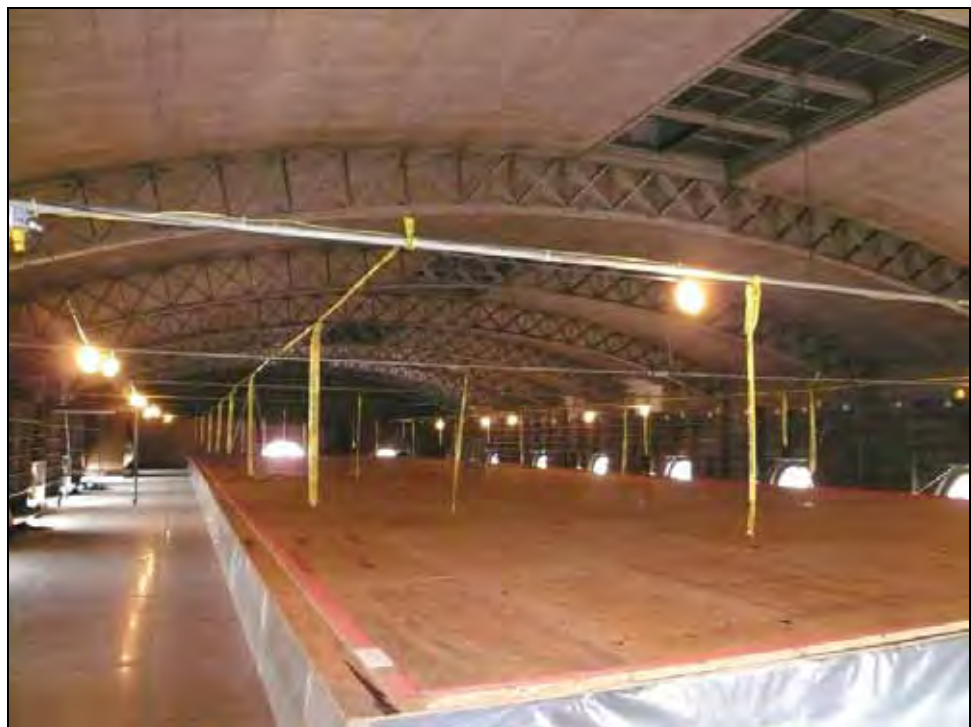
Figure 4: Exhibit Hall with temporary decking. Photo by M. Goeke, 2008
