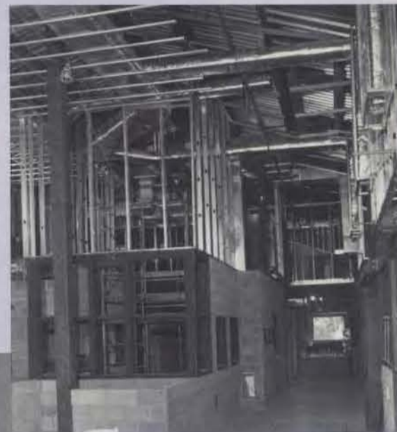
Interior of the building.
