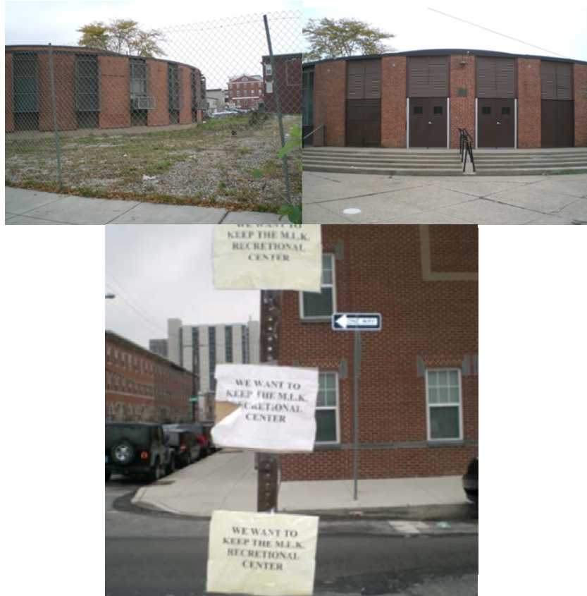
Figure 8: MLK Community Center from the side and back. Posted signs outside the building.
