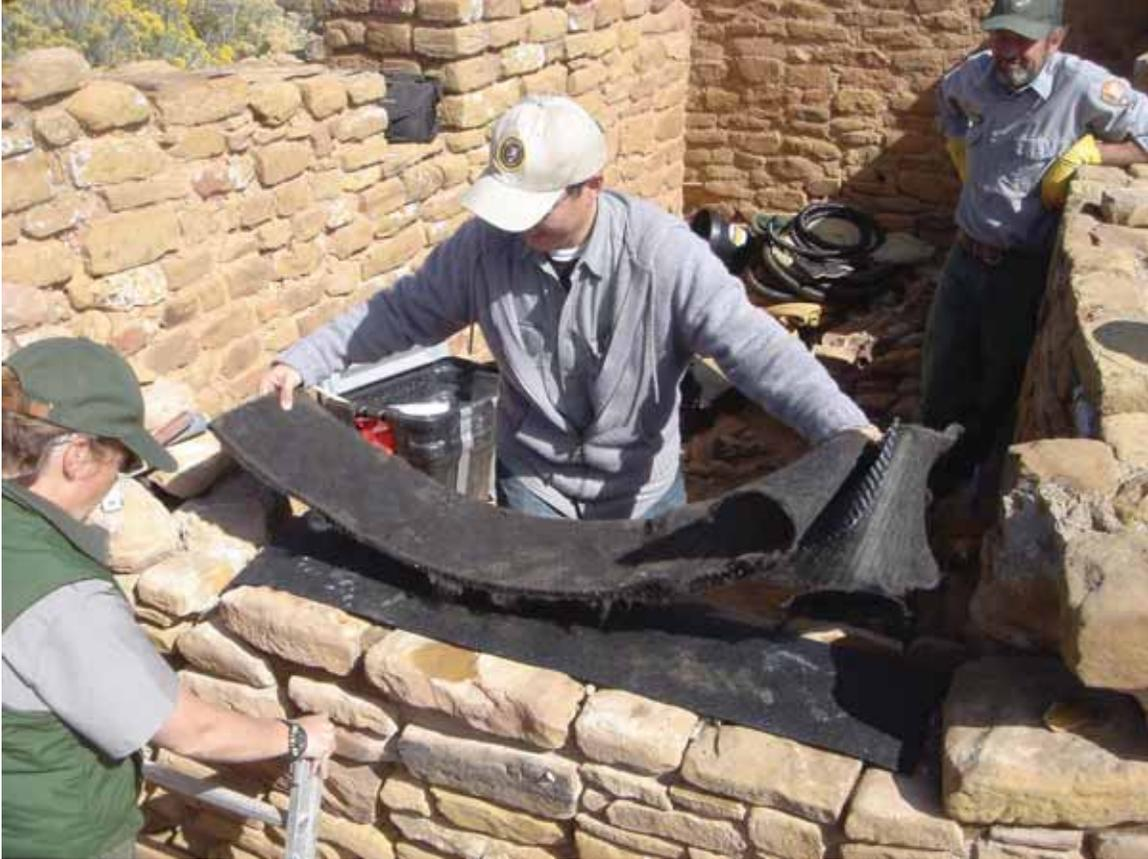
Figure 26. Geocomposite Installation (Matero 2008)
