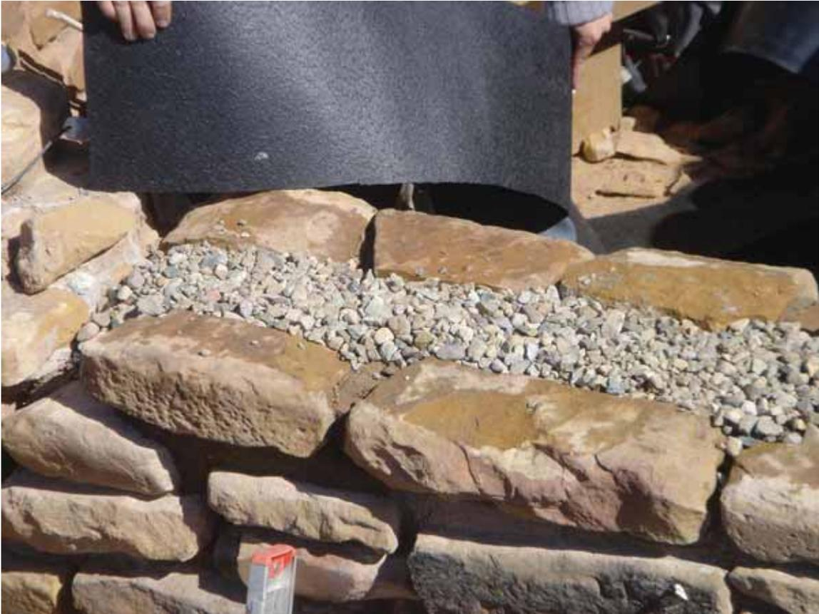
**Figure 25. Gravel Fill and HDPE Geomembrane Installation (Matero 2008)**
