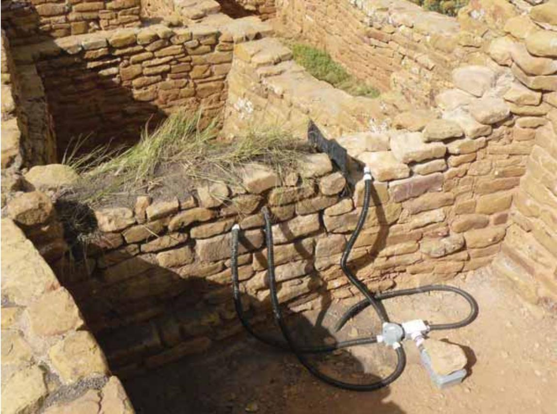
**Figure 29. Completed Moisture/Temperature Monitoring System on Soft Cap (Matero 2008)**
