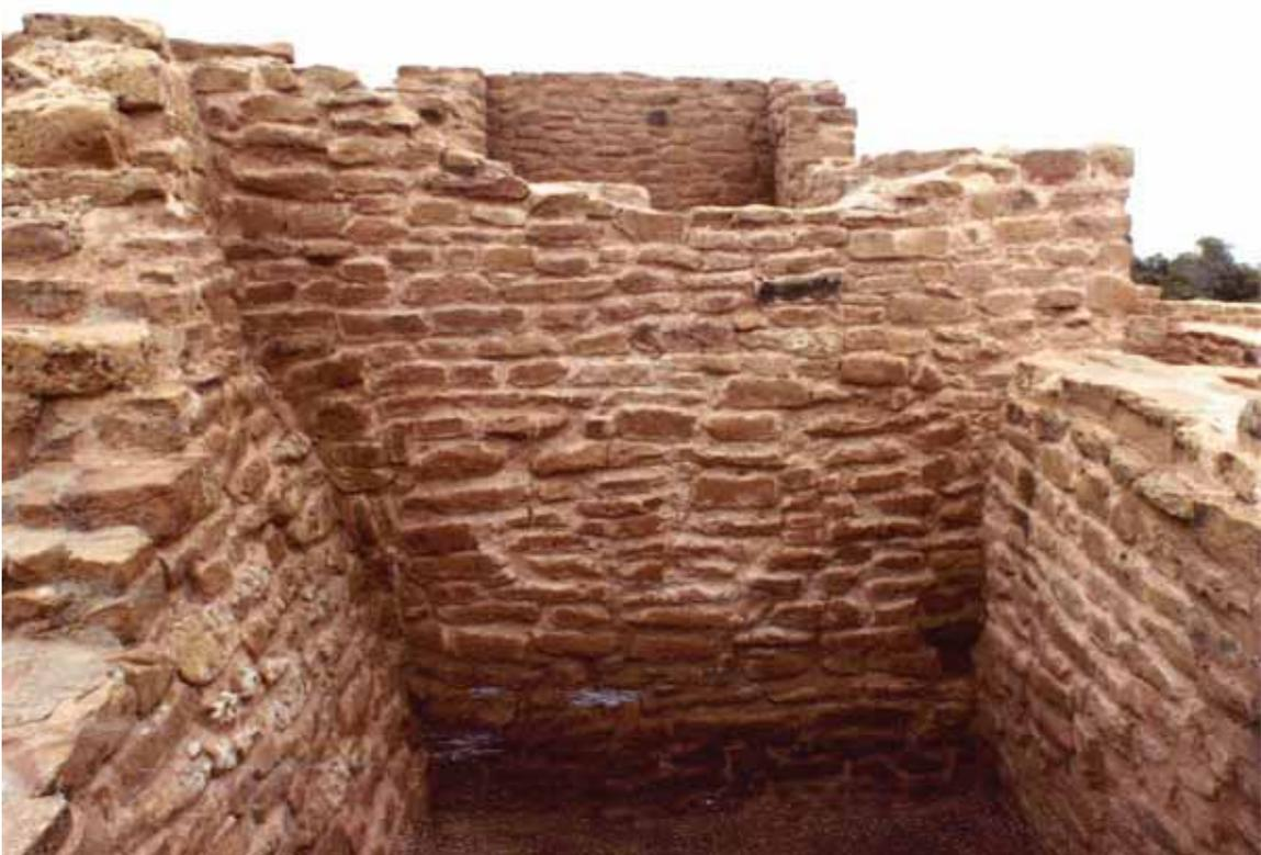
**Figure 18. Room 13 East Wall in 1983 after Re-Stabilization (Fiero 1983) MVRC**
