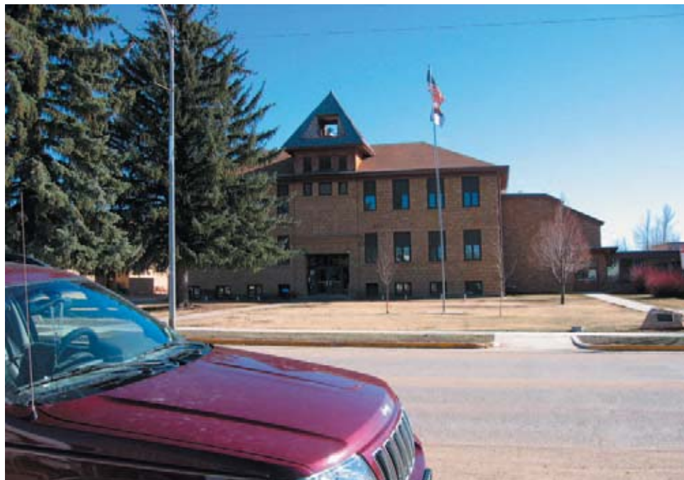
Figure 40-Mancos High School, Mancos, 2005
