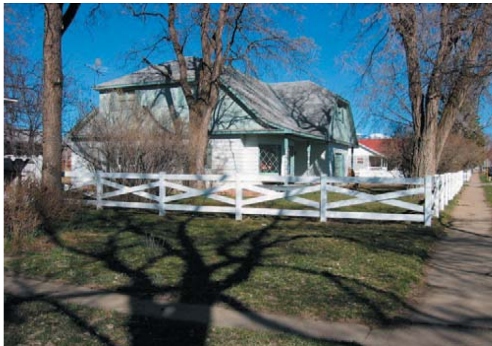
Figure 38-Preserved Residence on Grand Avenue, Mancos, 2005
