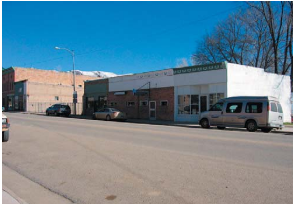
Figure 42-Buildings and Vacant Lot along Grand Avenue, Mancos, 2005
