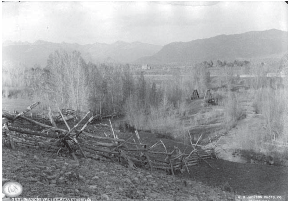
Figure 4-The Wetherill Ranch c. 1890 (Source: Denver Public Library)
