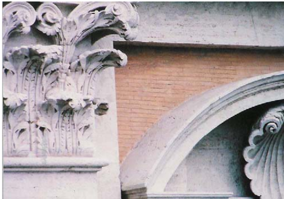
Figure 4.4: An example of travertine and cortina finishes used on the Capitoline Palaces, and a detail of the cortina finish (Sardegna, 2004)
