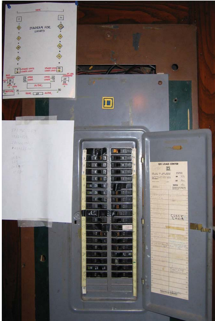
Figure 5: A circuit breaker panel in St. Agatha-St. James Roman Catholic Church in Philadelphia. Most of the luminaires in the church are controlled from this panel, but many are controlled from other isolated switches, including one located just above the floor in one of the side altar areas. Note the diagram to help make sense of which switches control which luminaires, and the electrician’s tape covering some of the switches as a way to keep them either always on or always off.
