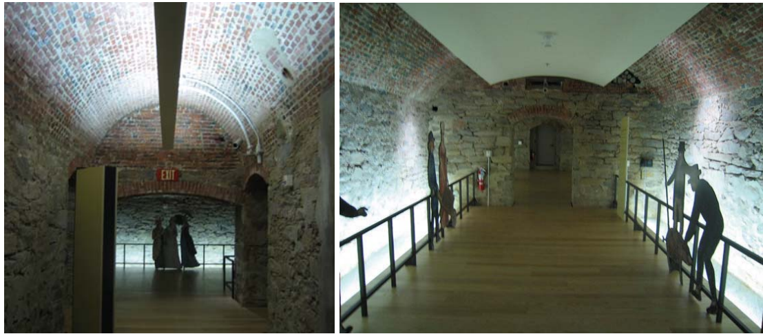
Figure 11: The basement level of the Second Bank of the United States in Philadelphia. The indirect and floor-mounted luminaires are unlikely to be mistaken for “historic” lighting.
