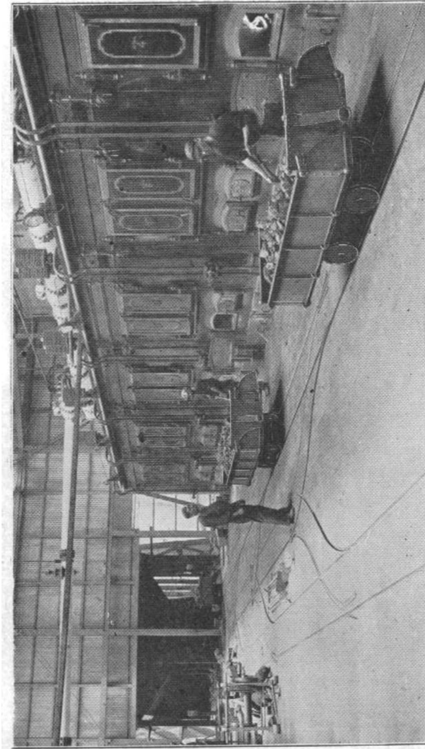
Figure 18: C.W. Hunt coal-charging miniature railway system for a power station. C.W. Hunt Company, No. 9306: Coal Handling Machinery . Staten Island, NY: C. W. Hunt Company, 1893, http://archive.org/details/coalhandlingmac00compgoog , 44.
