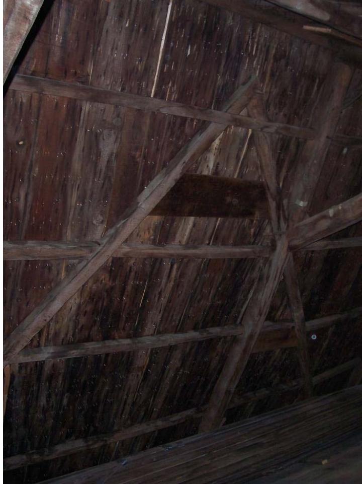
Figure 15: Remnant of the original 1680 structure in the Garrett, 2006.
