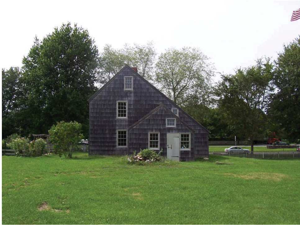
Figure 4: Eastern façade of Mulford House, 2006.
