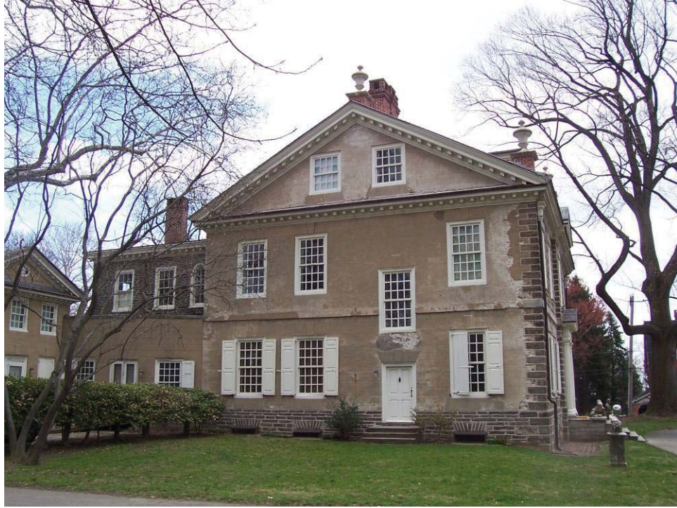
Figure 23: Northwestern façade of Cliveden, 2007.
