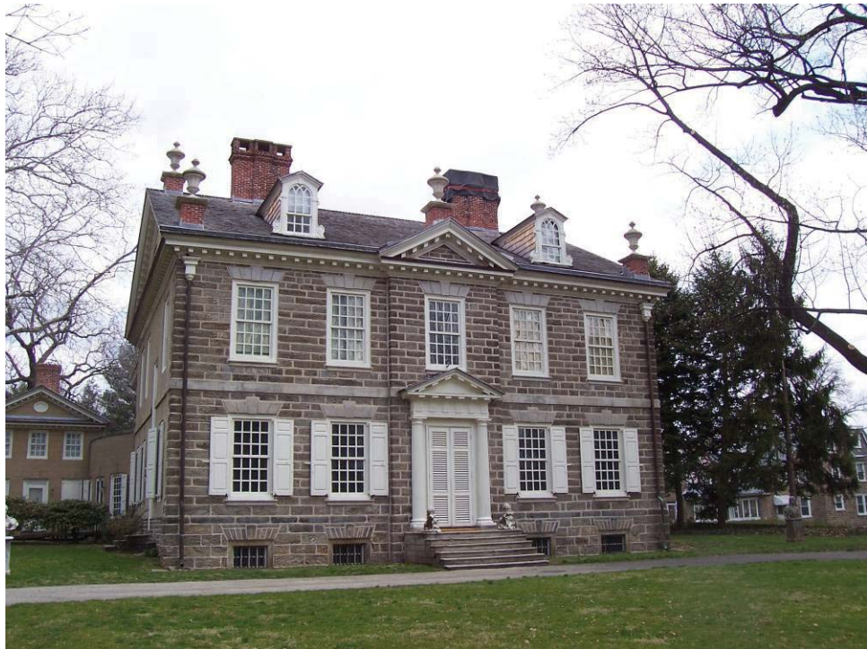
Figure 22: Front view of Cliveden, 2007.
