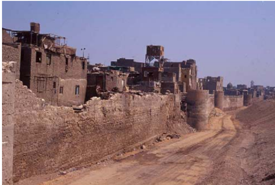
Figure 1.1: The eastern section of the Ayyubid wall during restoration (ACL).
