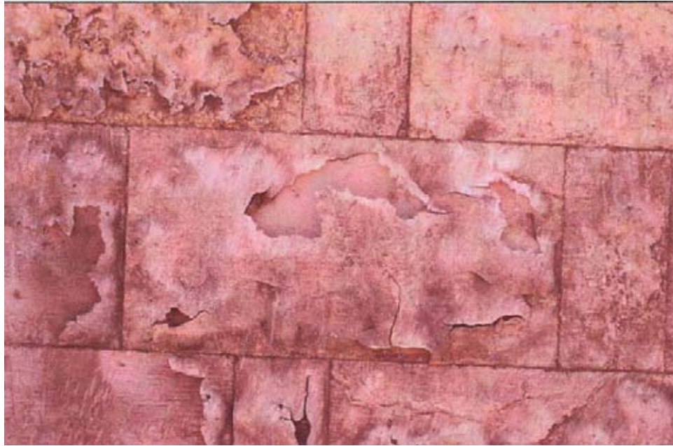
Figure 1.3: Detail of thin salt crusts on the surface of the Egyptian limestone in the wall (from Bourguignon).
