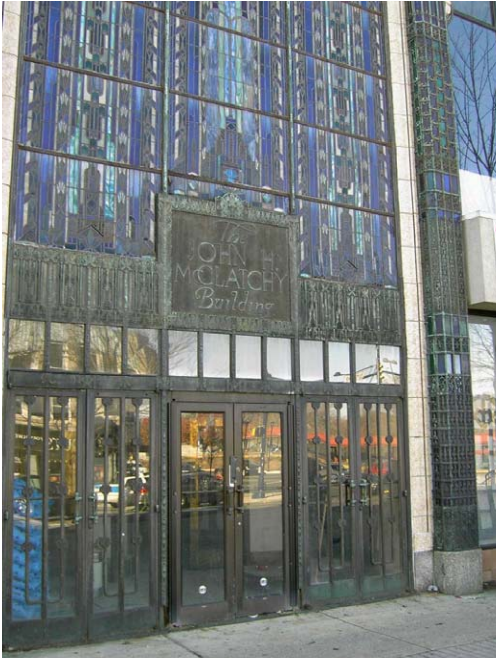
Figure 7. 69 th Street Entrance (photograph by author)
