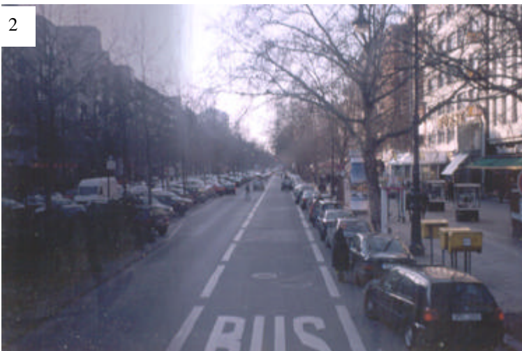
Bus lane: low investment cost and simple, but difficult to protect for buses only (Berlin)
