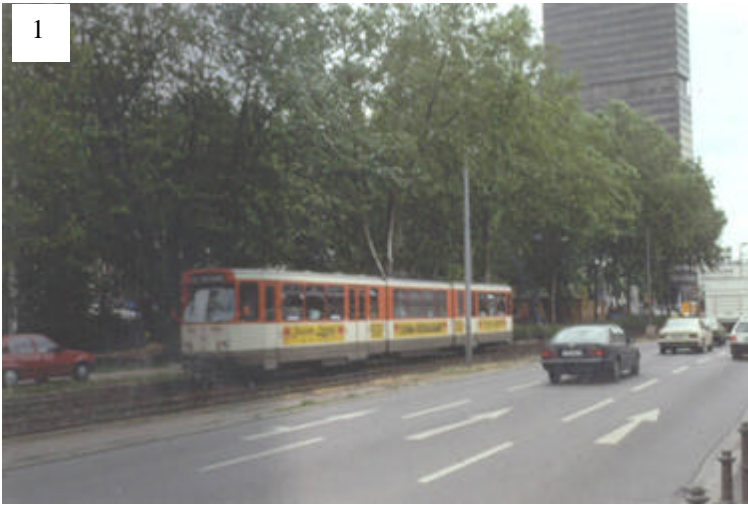
Typical LRT median ROW: distinctly separated from roadway (Frankfurt)
