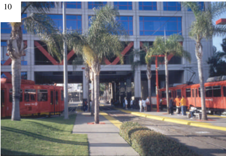
LRT integrated with office building in San Diego
