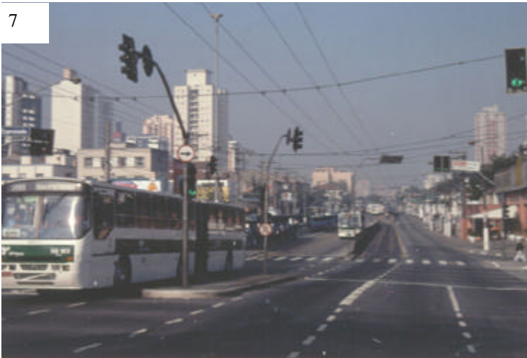
Hundreds of buses and trolleybuses per hour use this busway in Sao Paulo
