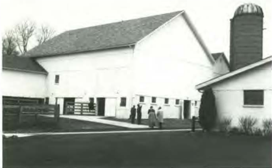
The Dorothy Russell Havemeyer Barn located at the Georgia and Philip Hofmann Research Center for Animal Reproduction at the School's New Bolton Center campus.
