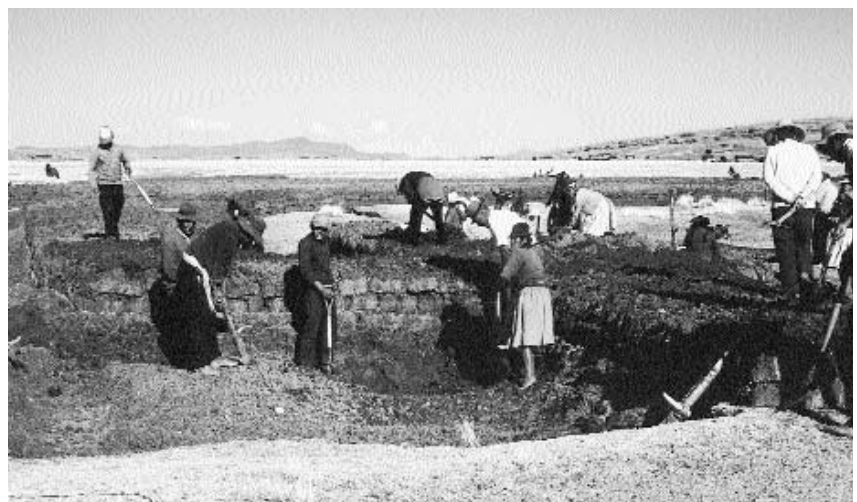
Figure 4 Construction of experimental raised fields during the dry season by farmers of Huatta, Peru, 1986. Photo provided by Instituto Geográfico Militar. (See also Color Plate 13.)
