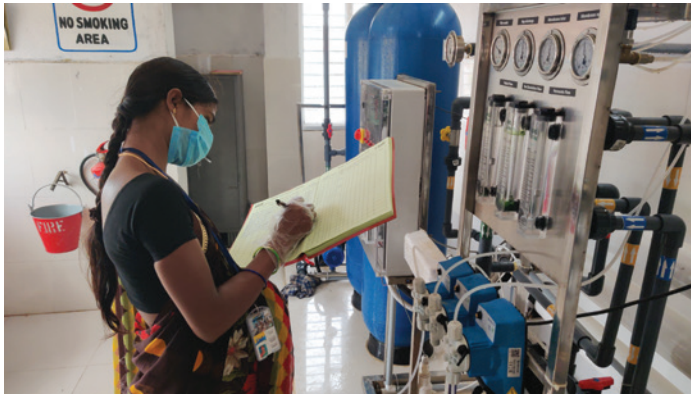
Figure 1: iJal (“Water ATM”) operator reviewing water flow parameters during a water plant visit. These data can also be accessed remotely to minimize on-site requirements, especially during COVID-19
