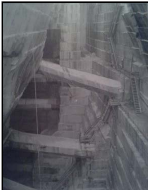
— Marble Quarry in West Rutland, Vermont (c. 1910s-20s)
