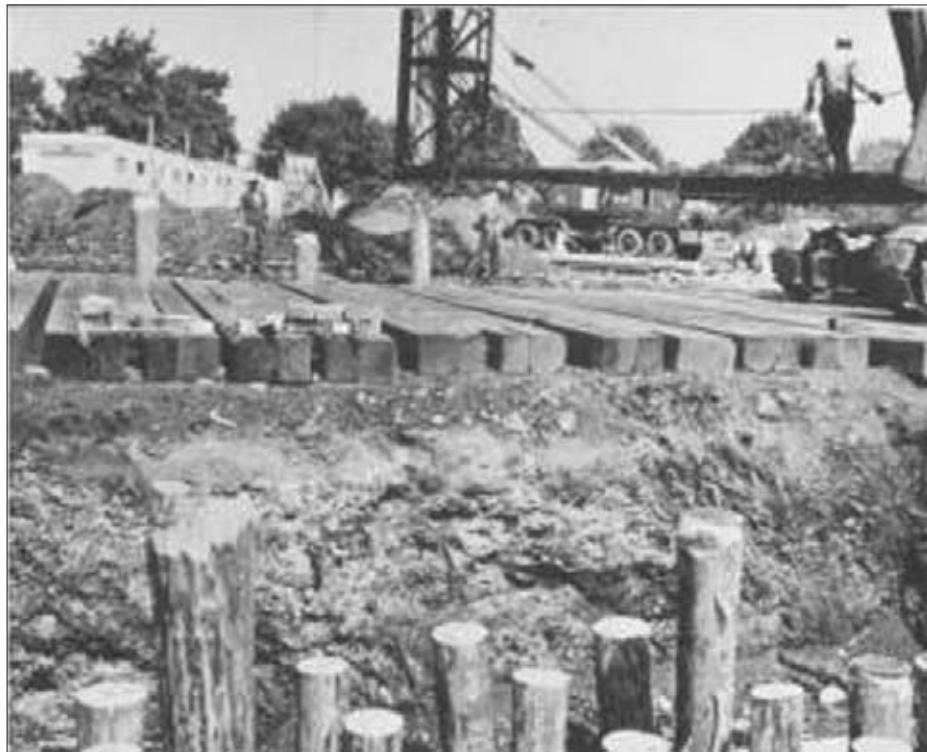
Figure 10 Wooden pilings, stacked and ready to be driven for Pavilion foundations.
