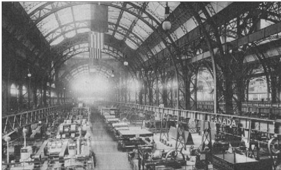
Figure 40 Interior view of Machinery Hall, showing exposed, internal structural steel frame (1893).
