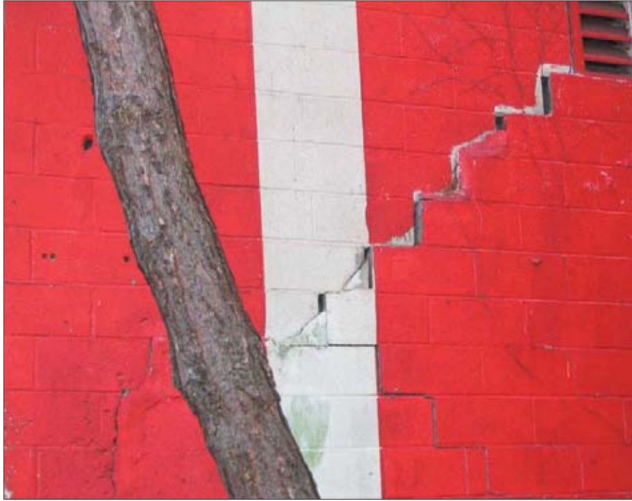
Figure 27 Typical severe step cracking at mortar joints of exterior CMU wall of one story perimeter structure.
