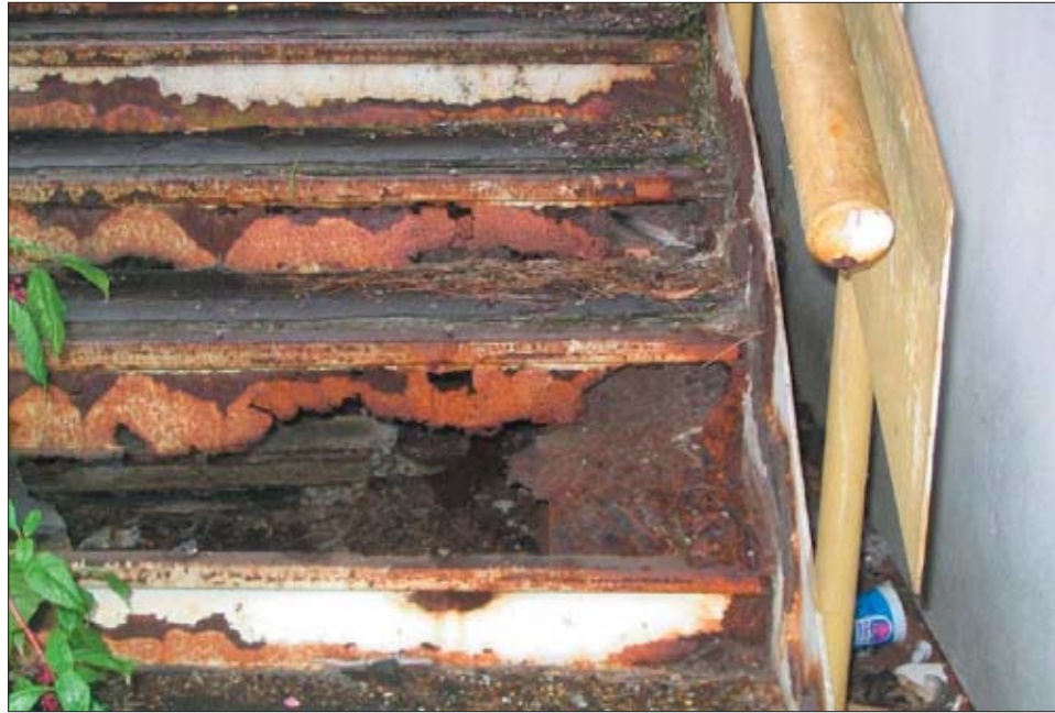
Figure 32 Typical deteriorated condition of interior stairs leading to promenade level.
