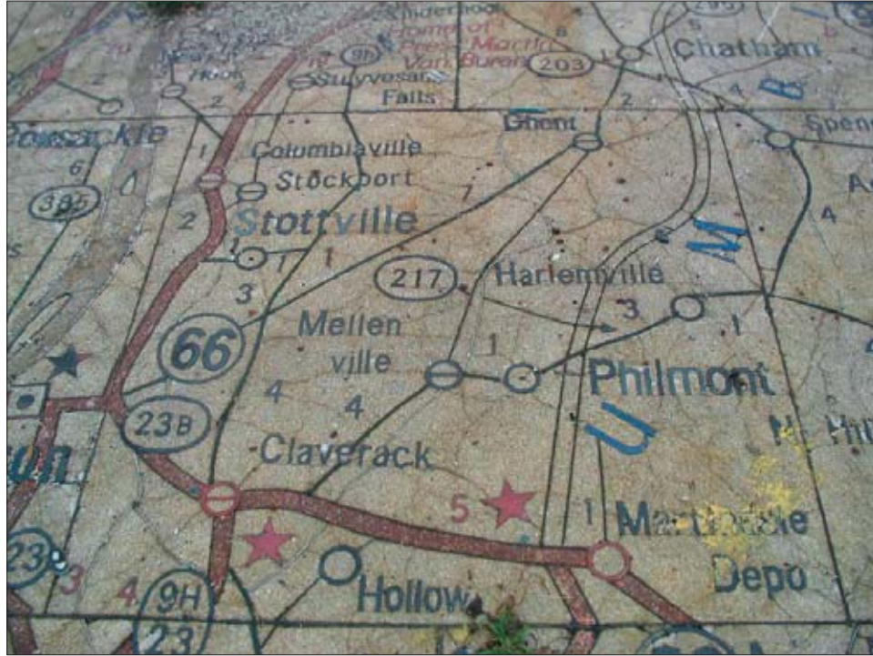
Figure 26 Close-up of the current terrazzo floor road map condition where vegetation has been cleared. Note extensive cracking.
