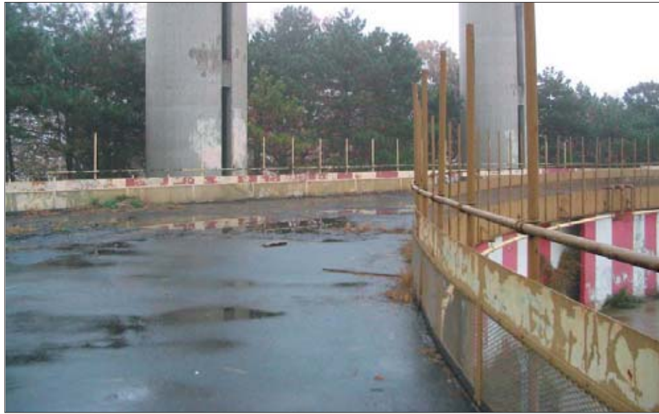
Figure 28 Condition at promenade level. Note uneven floor surface, ponding water and corroding steel railings.
