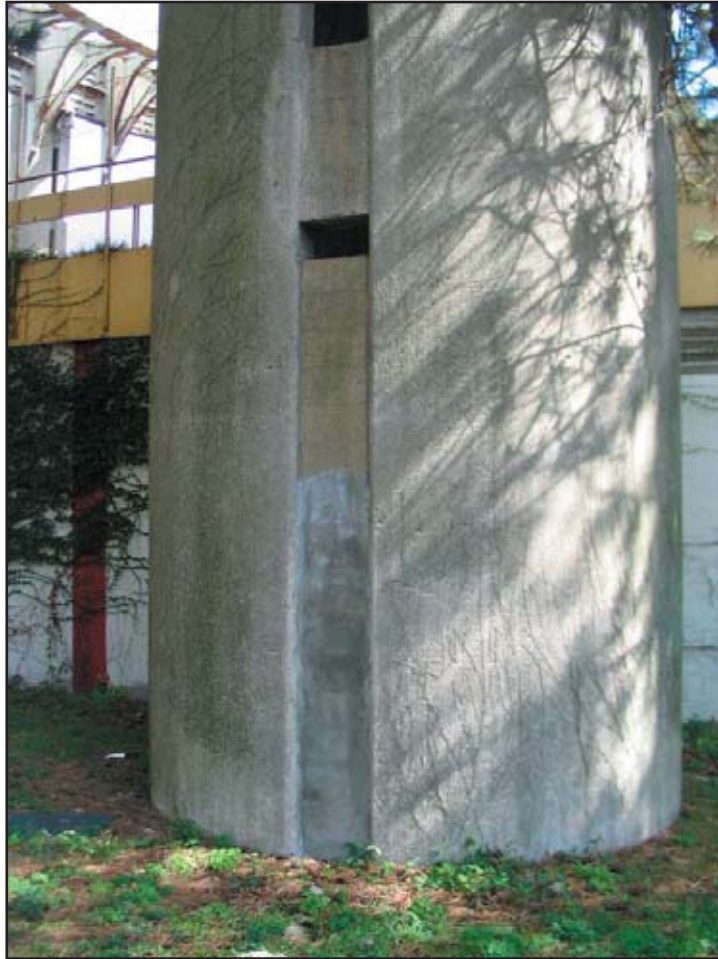
Figure 29 Typical Tent of Tomorrow column base, with CMU blocks filling opening to prevent entry.
