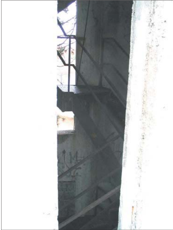
Figure 33 View of interior of Tent column with stairwell. Note missing stair treads.
