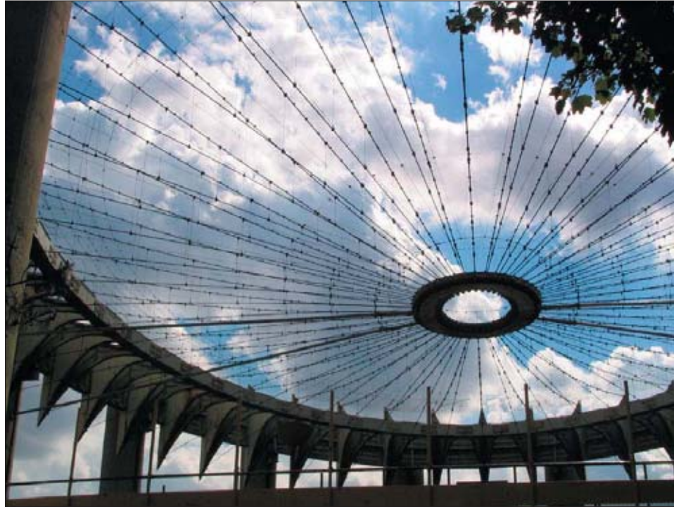
Figure 30 Bare bicycle wheel roof structural skeleton without original panels, exposing two layers of steel roof cables as well as steel compression and tension rings.
