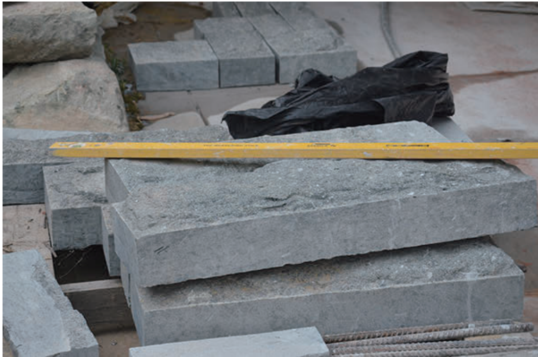
Figure 55. Replacement green granite panels are tooled on the surface to resemble natural stone. (August 2015, stfrancisparish.org)
