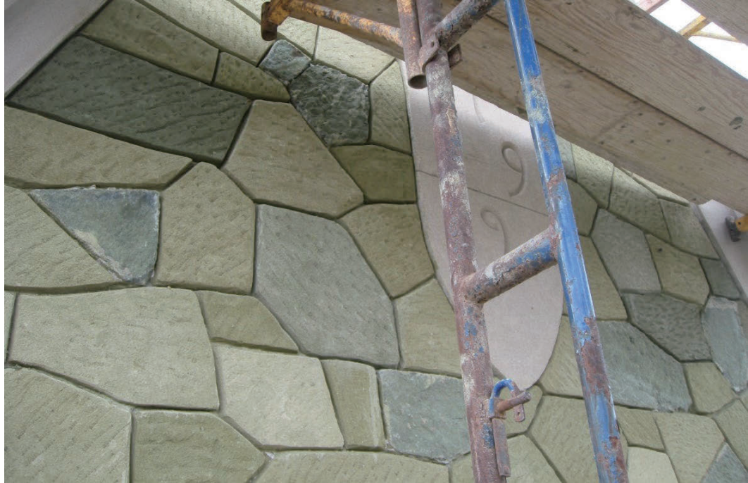
Figure 49. New face recreated with composite repair mortar. The joints were later pointed with Type O mortar. (Courtesy of Caretti Restoration & Preservation Services, L.L.C., 2011)
