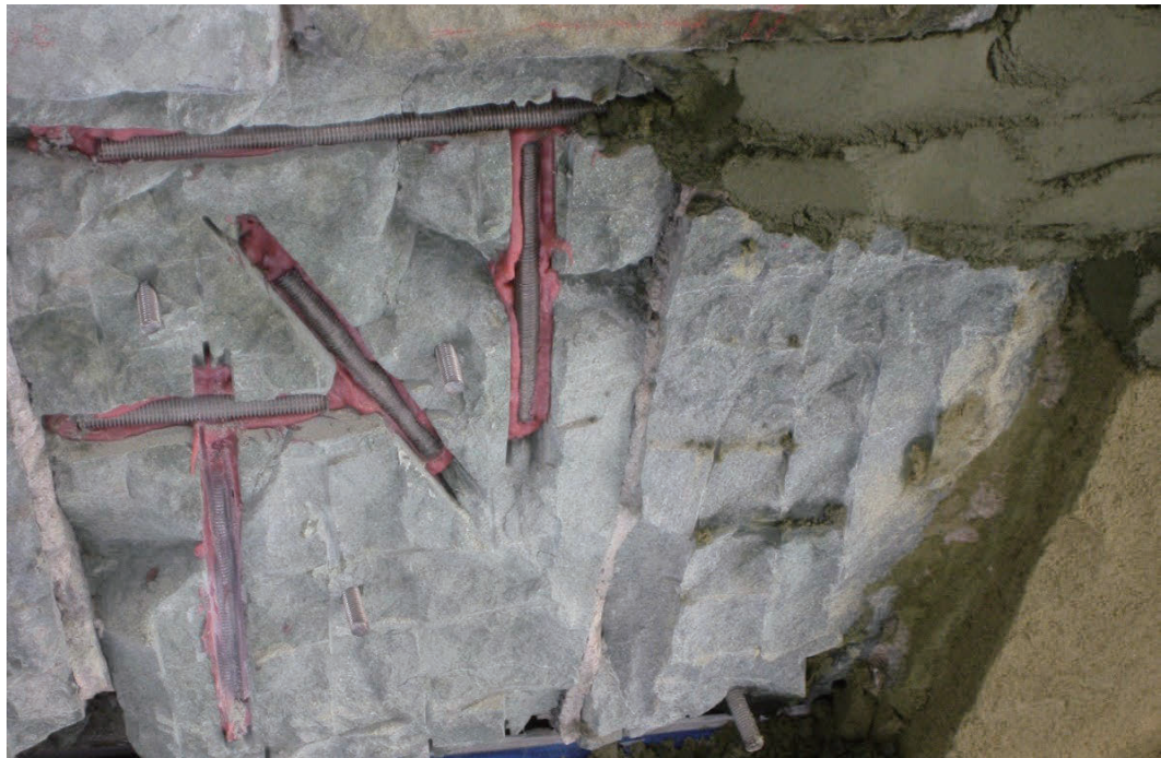
Figure 50. Stainless steel pins embedded in epoxy were used to provide additional support to keep the composite repair mortar in place. (Courtesy of Caretti Restoration & Preservation Services, L.L.C., 2011)
