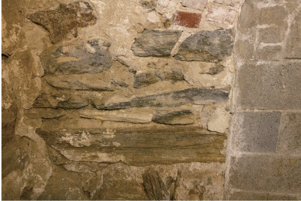
Figure 42. Section of exposed wall in the basement of Recitation Hall showing different types of stone, bricks, and concrete blocks. (Photograph by author, 2019)
