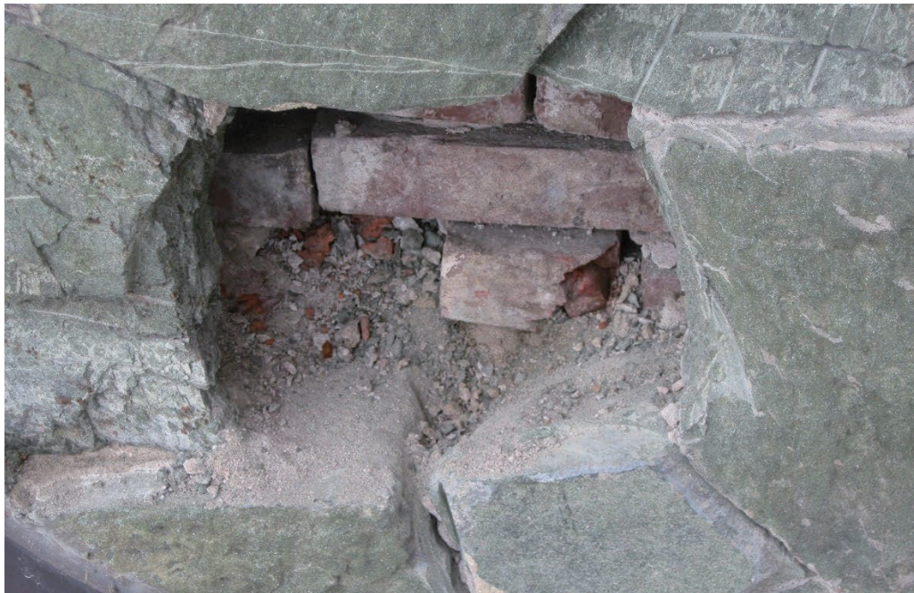
Figure 41. Parts of the back-up masonry were infilled with brick; it is not known if they are original or from subsequent repairs. (Courtesy of Caretti Restoration & Preservation Services, L.L.C., 2011)
