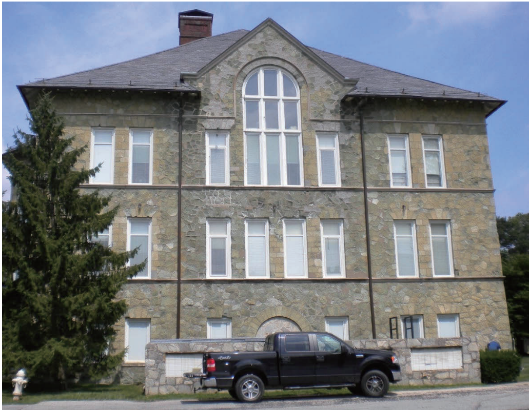
Figure 43. Pre-construction photograph of east elevation, Recitation Hall. Note the deteriorated stones below the third story window sills and on the gable. (Courtesy of Caretti Restoration & Preservation Services, L.L.C., 2010)
