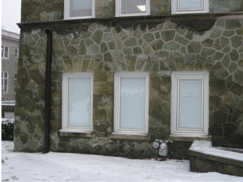
Figure 44. Stone underneath window sills are generally in worse condition. Note the dark stains formed from moisture accumulation. (Courtesy of Caretti Restoration & Preservation Services, L.L.C., 2009)
