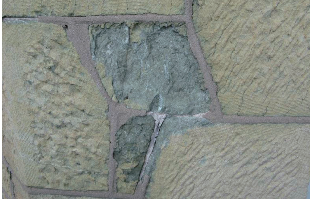
Figure 45. Detail photography showing the yellow crust on top of the serpentine, retaining its original tooling. The green stone has largely lost the crust with some remaining on the edges, it shows visible signs of erosion. (Courtesy of Schnabel Conservation L.L.C, 2008)
