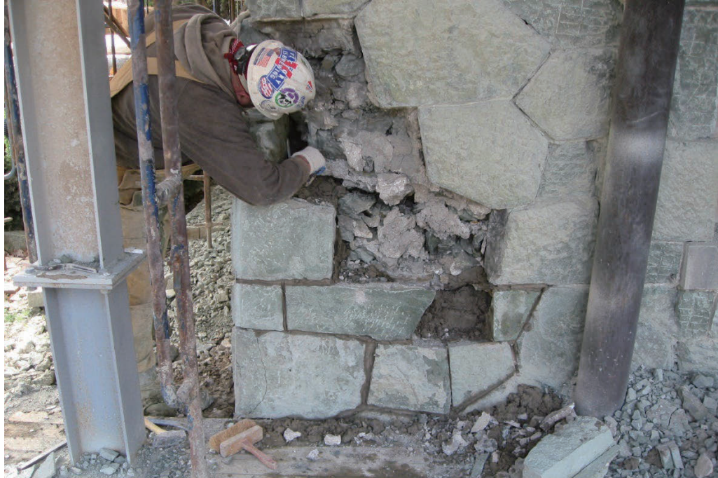
Figure 40. Exposed back-up rubble masonry wall during the repair campaign. (Courtesy of Caretti Restoration & Preservation Services, L.L.C., 2011)
