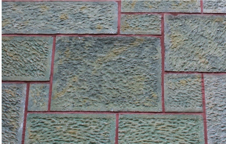
Figure 30. Detail of cast-stone with recreated original tooling. (Photograph by author, 2019)
