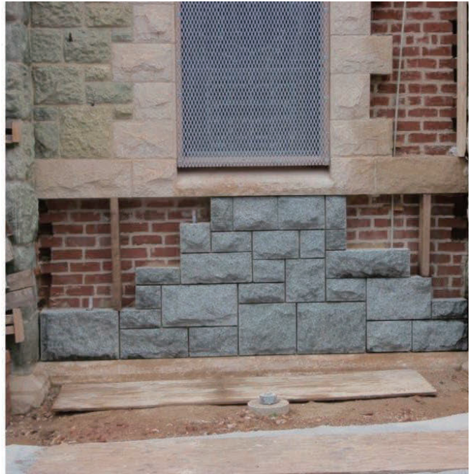
Figure 56. Left: drawing showing the numbered stone and its layout. Right: replacement green granite laid according to the shop drawing with the reconstructed brick wythe behind it. (wdpa.com)
