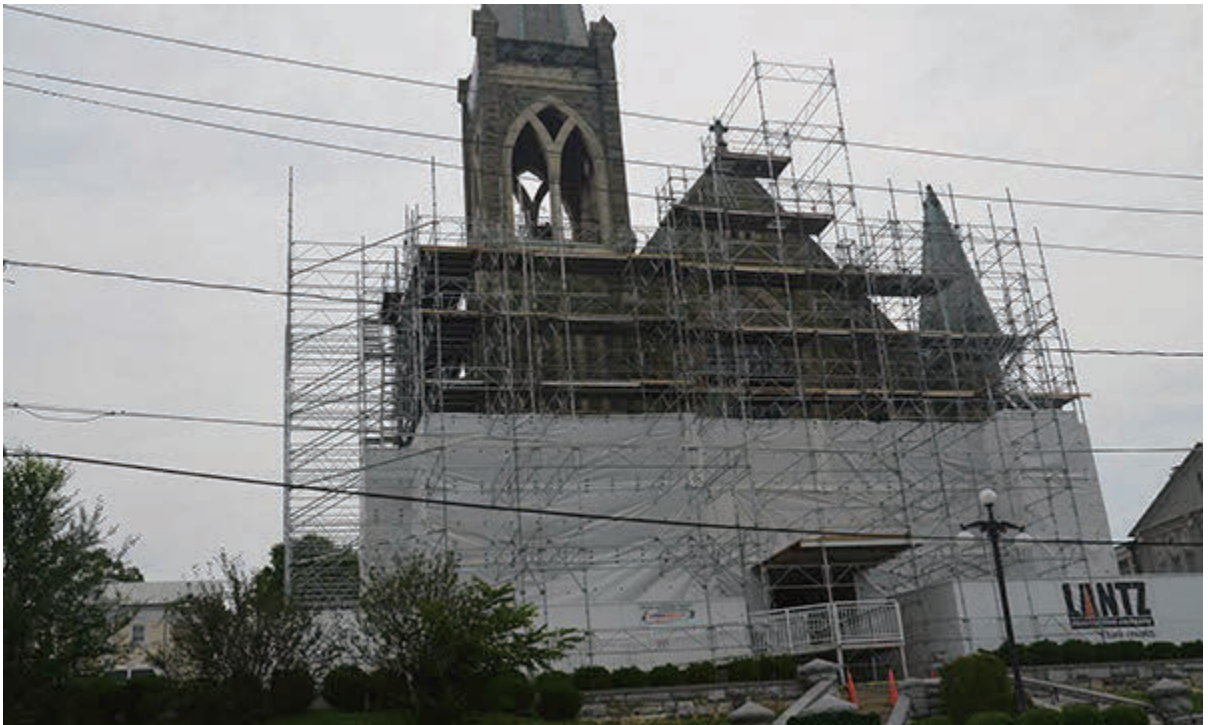
Figure 57. Scaffolding around the church were designed to allow entry to the church during construction. The plastic covering serve as weather protection and safety precaution. (July 2015, stfrancisparish.org)
