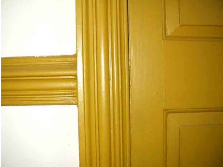
Above, Door Casing and Chair Rail, Below, Baseboard
