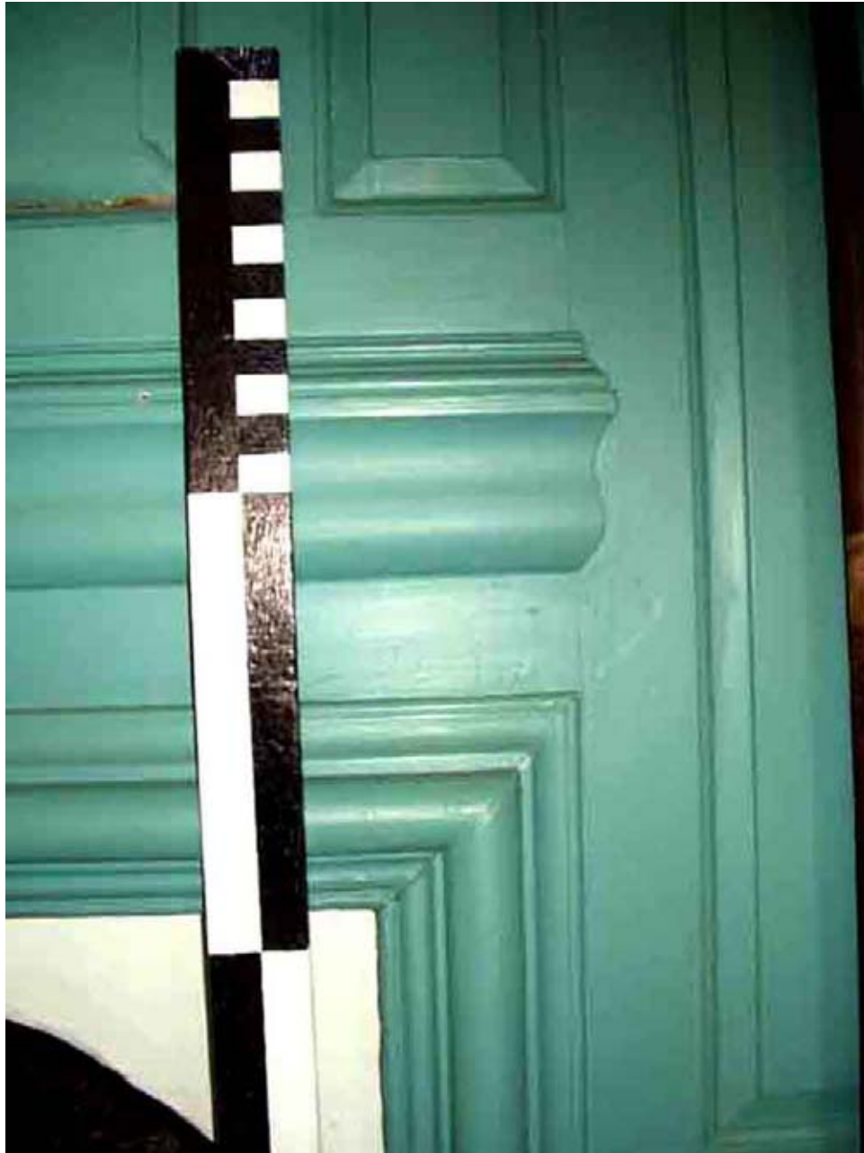
Fireplace Overmantel and Bolection Molding Detail
