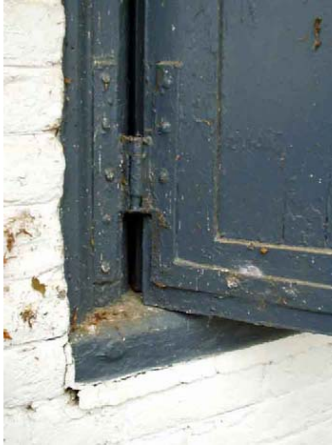
Shutter H-L Hinge Detail
