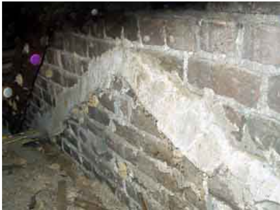
Above, Kitchen Roof Rafters. Below, Scar From Original Kitchen Roof on Main Block's East Façade.
