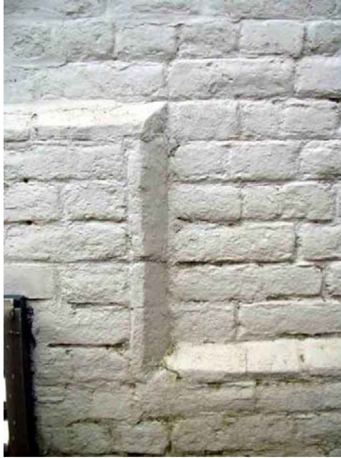
Chamfered Watertable Jog Over Cellar Window
