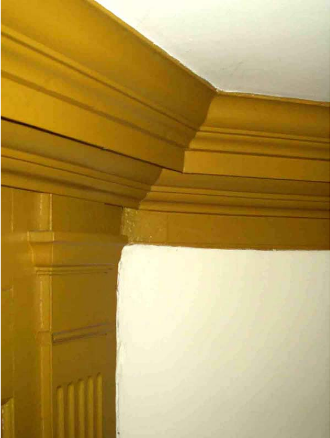
Cornice and Pilaster Detail
