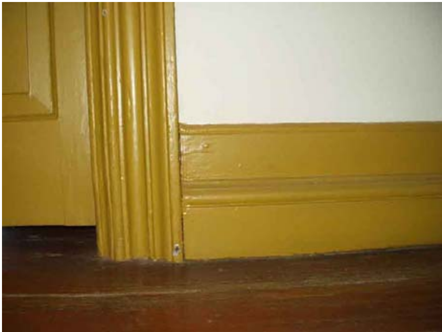
Above, Door Casing and Chair Rail, Below, Baseboard
