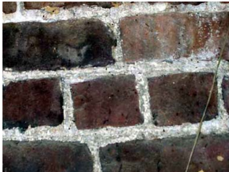
English Bond Brickwork Detail, East Gable End
