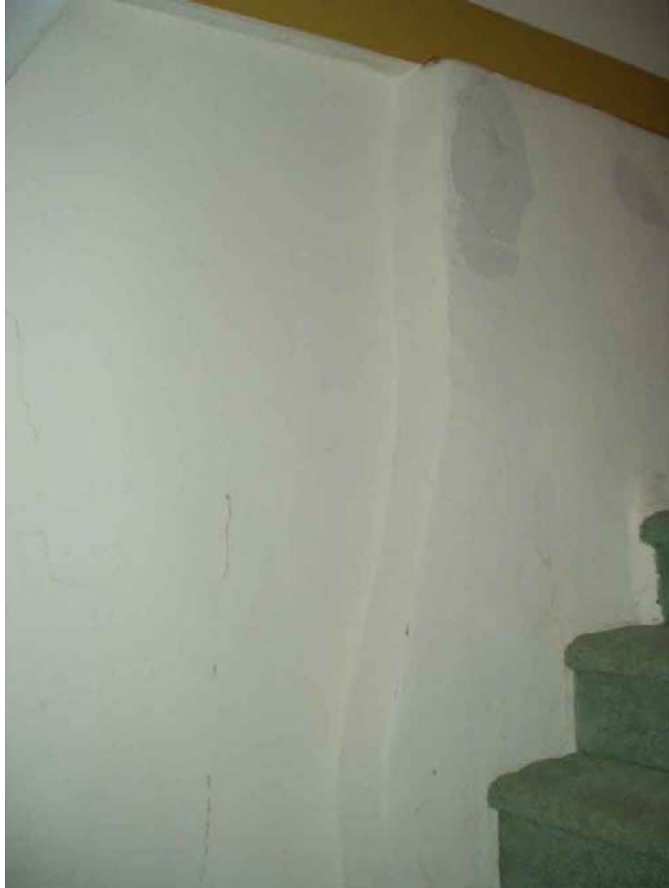
North Kitchen Stair Hall, East Wall Fireplace Chimney Scar.
