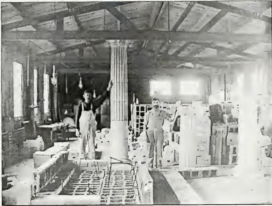
Figure 6: This photo shows terra cotta blocks being arranged in sequence and numbered to ensure proper installation on-site. Image found in the Ketcham Collection at the Athenaeum of Philadelphia.
