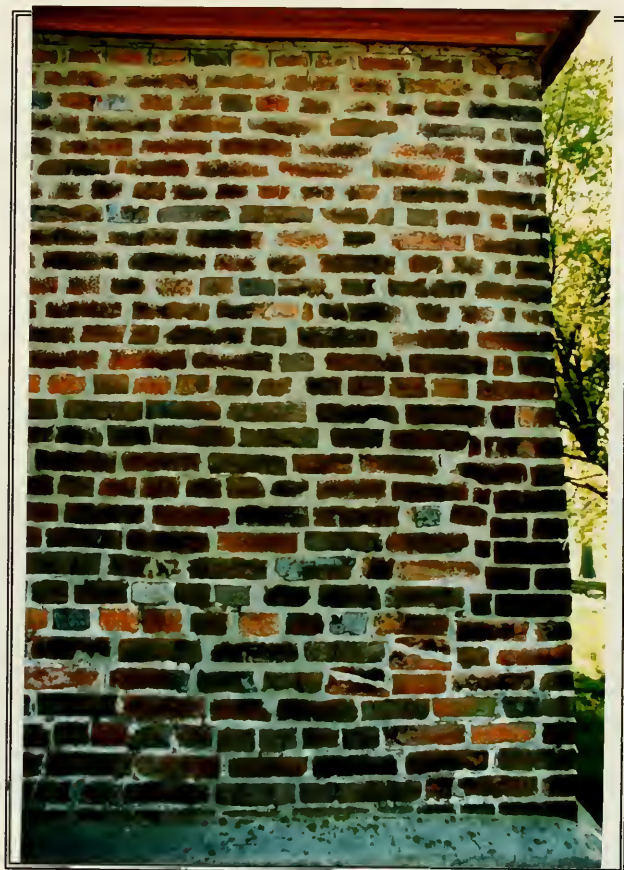
Figure 43. Disturbance in brick, kitchen, north elevation.
