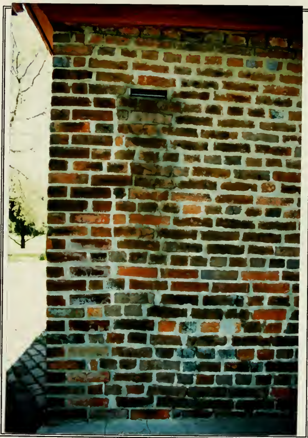
Figure 42. Disturbance seam, kitchen, north elevation.
