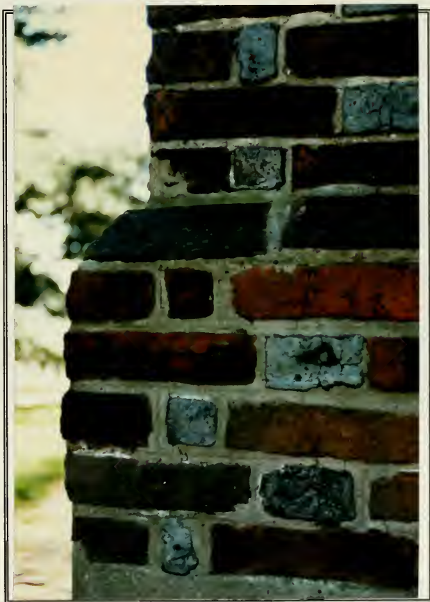
Figure 10. Water table, northeast corner.
