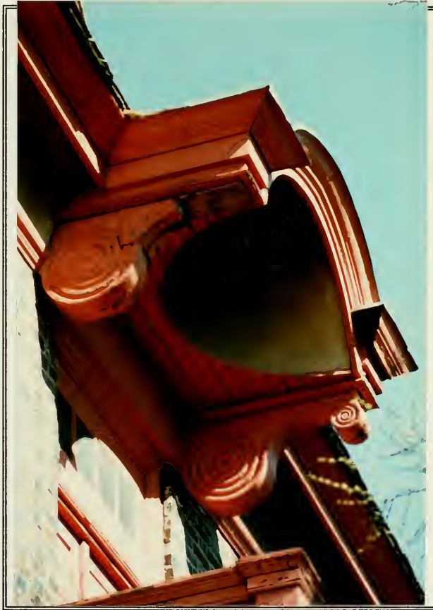
Figure 20. Coved hood, south facade, second floor, bay 3.
