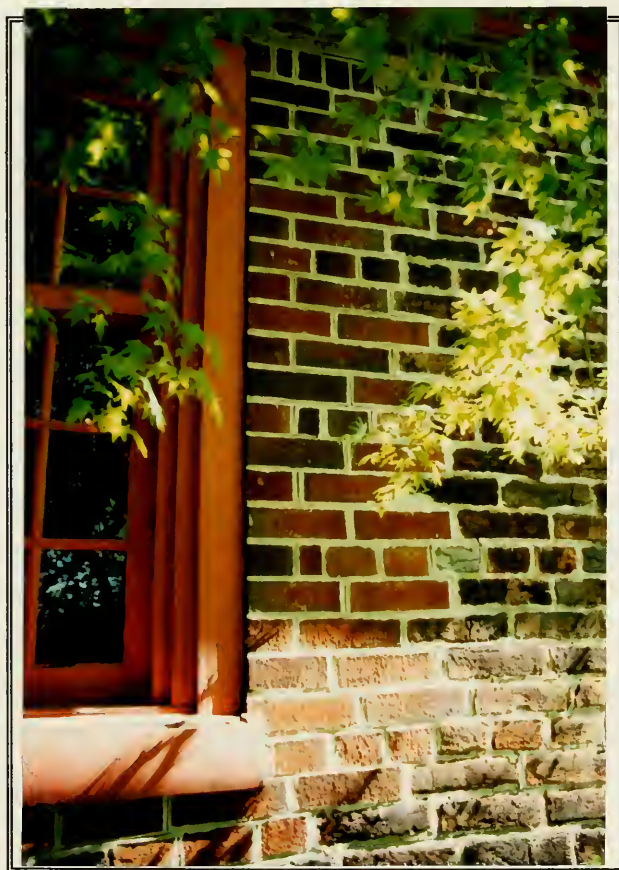
Figure 39. Detail of brick disturbance, kitchen, west elevation.
