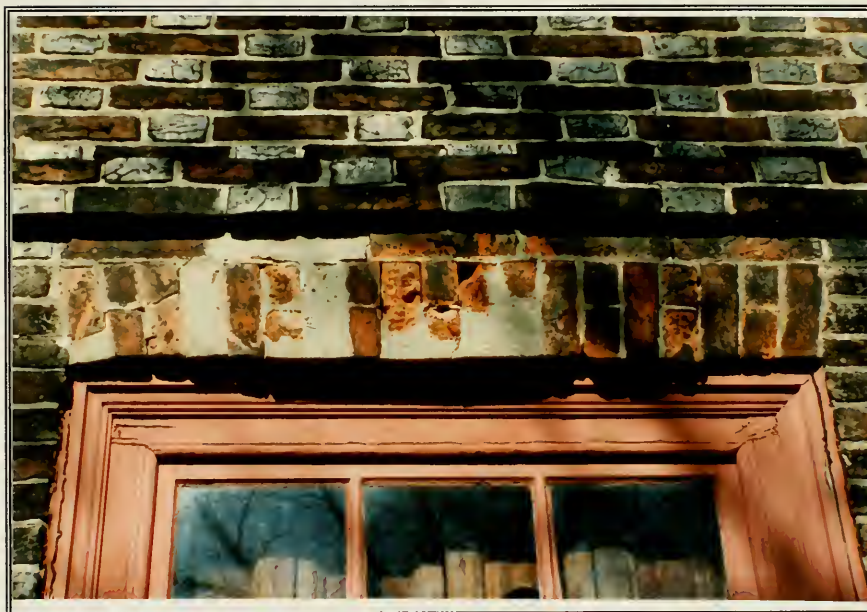
Figure 15. Jack arch above window, south facade, first floor, bay 1.
