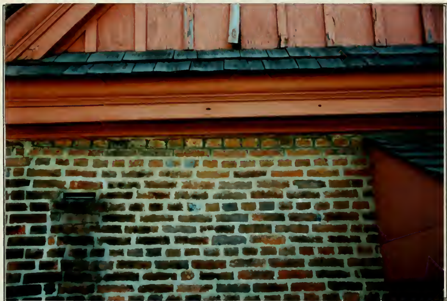
Figure 41. Detail, brick disturbance below roof line, kitchen, north elevation.
