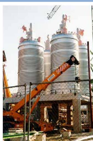
4 reactors 110 m 3 3 stages of GlasLock® agitators
