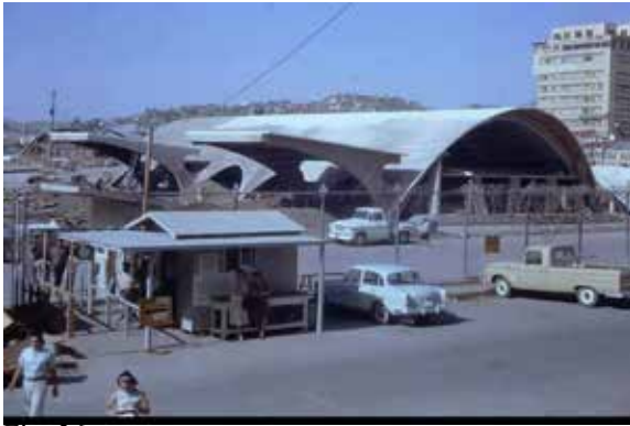
Fig. 36 Parking area with cantilivered canopies during construction. Source: Nogales de mis recuerdos
