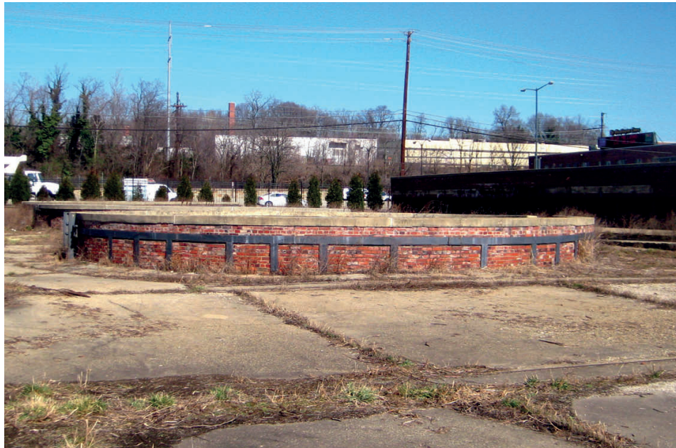
Figure 3.19: Preserved remains of a United Clay Brickworks beehive kiln. Courtesy of Author, 2012.
