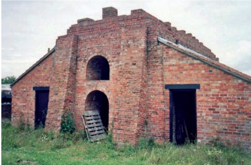
Figure 2.14: Modified version of a Scotch Kiln. "Baumber Brick Kiln." Ken Redmore, photographer, 2006. Society for Lincolnshier History and Archaeology. Image from http://slha.org.uk/slha/Main/GalleryBricks .
