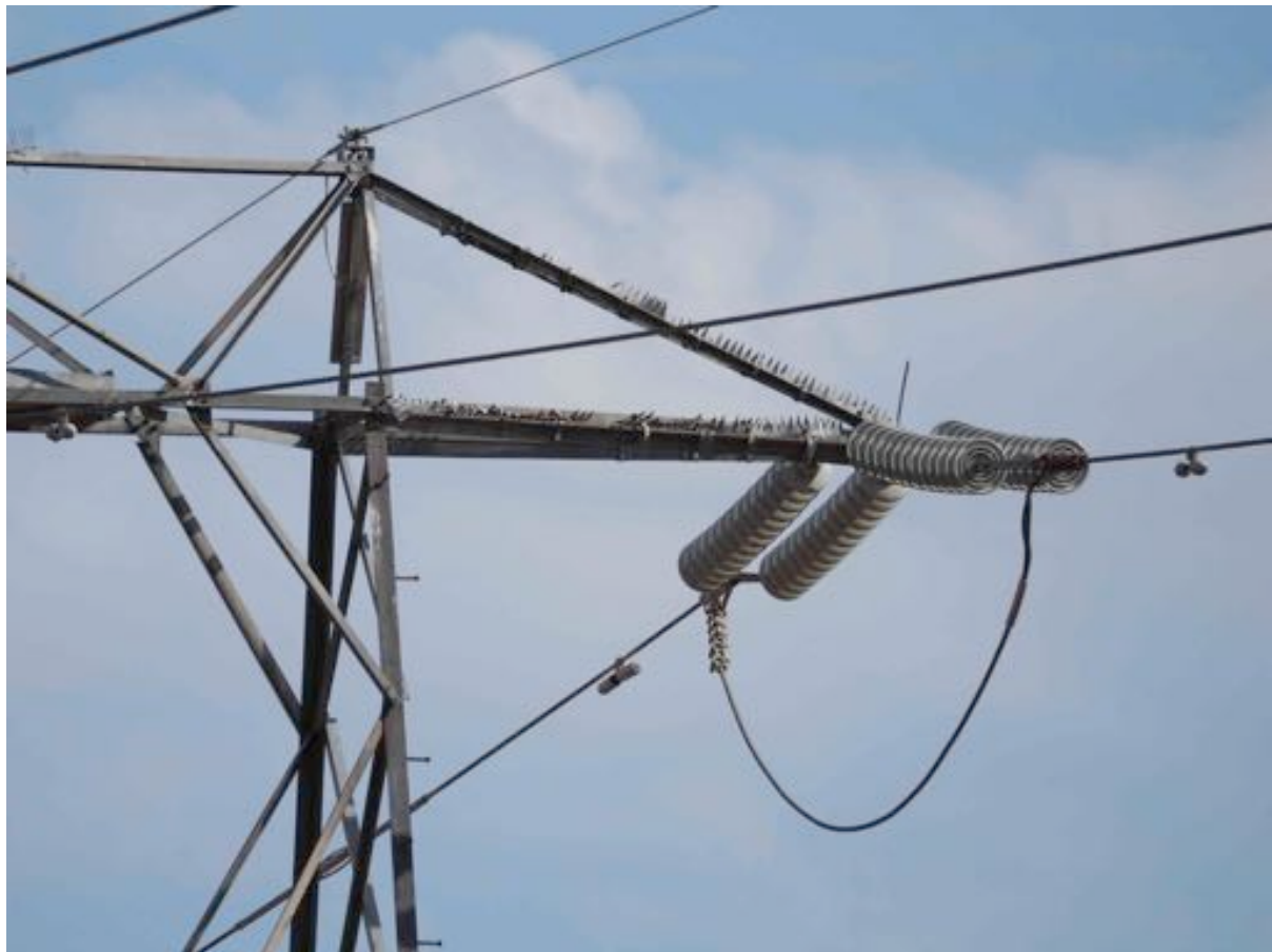
Figure 4. Spikes on the outer crossarms of one of the Big Creek transmission towers in the Central Valley of the kind that were first installed in 1924. The edge of a horizontal steel pan meant to catch bird excrement can be seen at the left. The smaller spikes on the crossbar above the central wire at the upper left of the image are a more recent innovation. Photograph by author.
