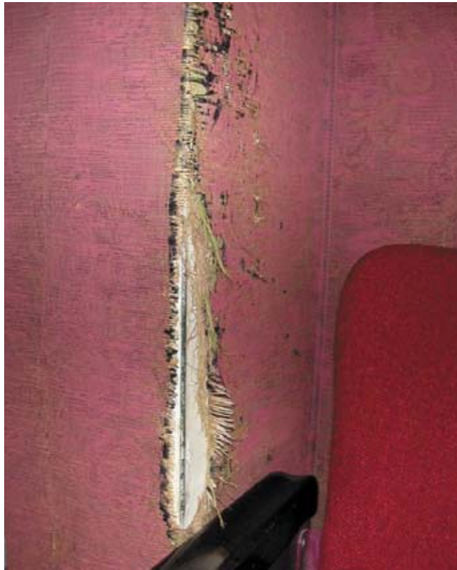
Fig. 46, Above , Fabric Pulling Away from Wall
