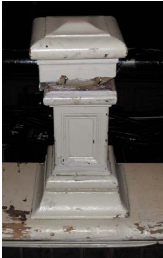
Fig. 41, Left , Damaged Balcony Post
