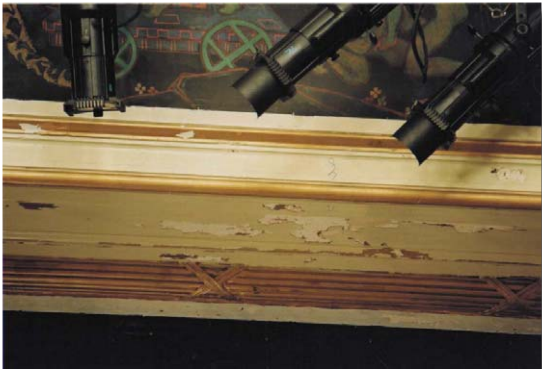
Fig. 36, Chipping Paint on the Proscenium
