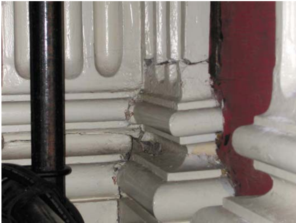
Fig. 39, Horizontal Cracking at Pilaster Bases
