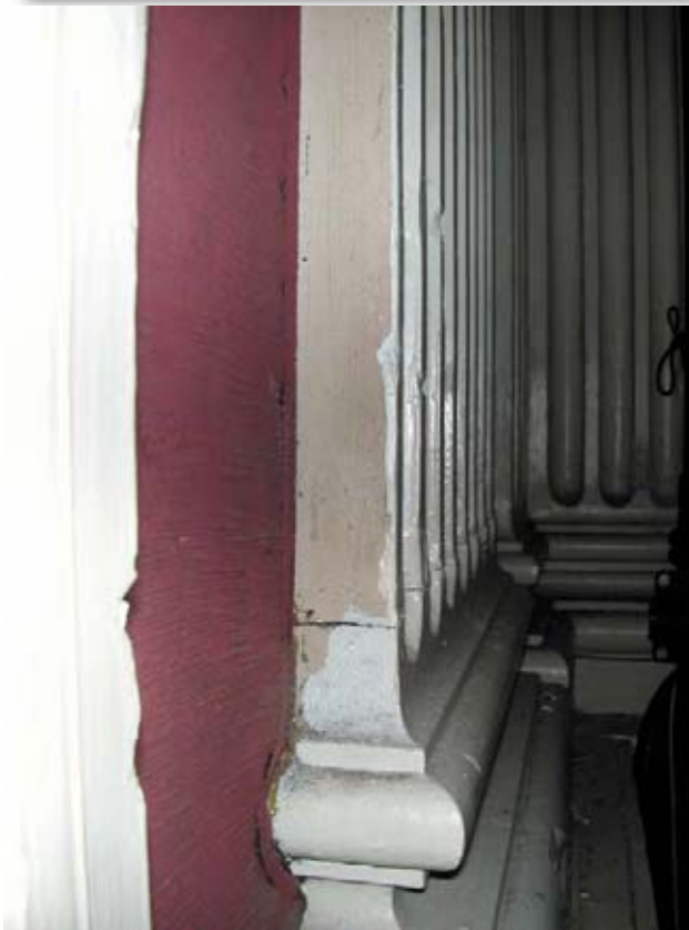
Fig. 32, Above , Pilaster Base with Chipped Paint
