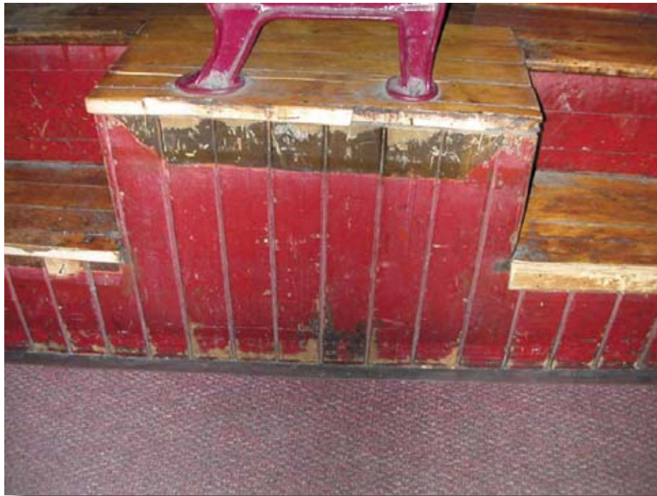
Fig. 29, Above , Chipping Red Paint on Seating Platfroms Fig. 30, Below , Moulding Missing from Seating Platform
