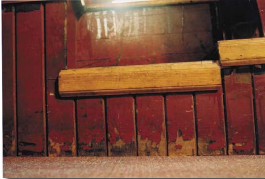
Fig. 29, Above , Chipping Red Paint on Seating Platfroms Fig. 30, Below , Moulding Missing from Seating Platform
