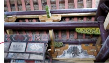
Figure 2.7m Shunshenchuan and the bracket set atop, Pingxianglou
