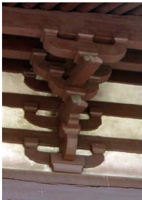
Figure 1.2i Front view of intercolumnar set, Main Hall of Tianningsi
