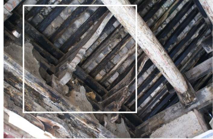
Figure 2.11e Picture of the rear view of the intercolumnar set, the Main Hall, Dubaisi
