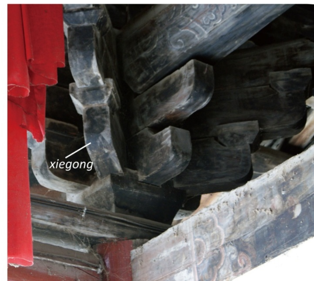
Figure 2.10d Picture of the rear view of the capital set, Main Hall, Dou-Kousi
