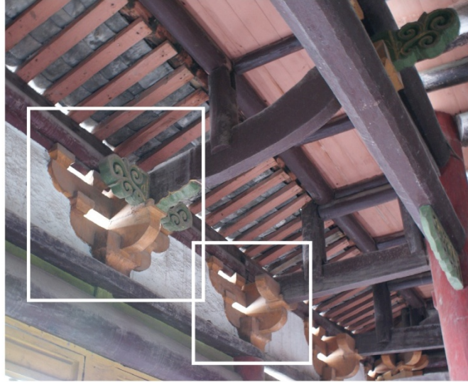
Figure 2.7f Picture of an intercolumnar set(left) and a capital set(right) from inside, Pingxianglou
