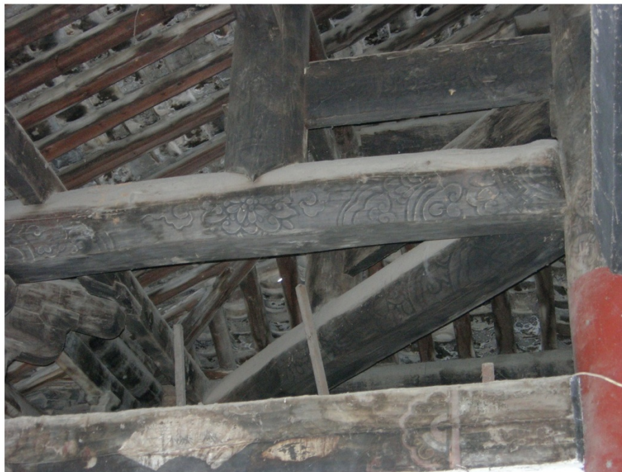
Figure 2.10h Color paintings on the components and the pointed bottom of the dwarf pillar, Main hall, Dou-Kousi
