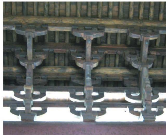
Figure 1.1k Picture of the rear view of intercolumnar set, Main Hall, Yanfusi
