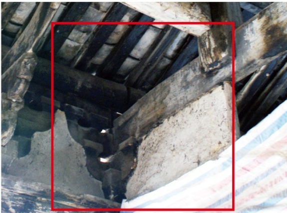
Figure 2.11f Picture of the rear view of the capital set, the Main Hall, Dubaisi
