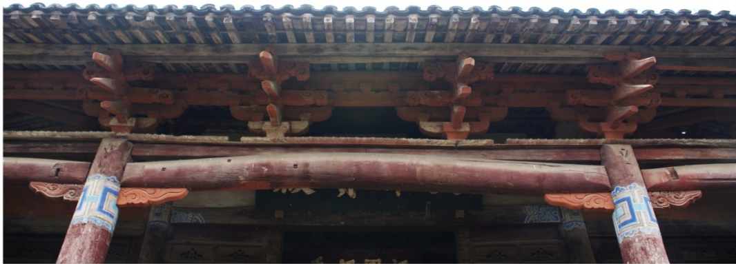
Figure 2.4e Capital Sets and Inter-columnar Sets in the Mingjian on the facade, Main Hall, Yong'ansi
