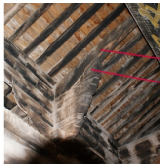
Figure 2.5e Rear view of the intercolumnar set, Wenchangdian, Wulongmiao
