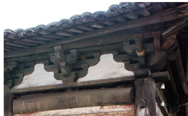
Figure 2.6d Corner set and intercolumnar set in the cijian , Main Hall, Qinglongsi
