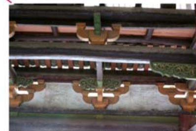
Figure 2.7o Curved traversal tie beam and the bracket set atop,
