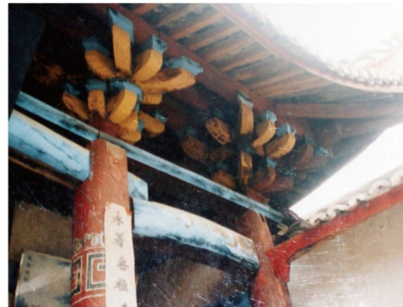
Figure 2.9h Picture of the capital and corner bracket sets, Yong'anmiao
