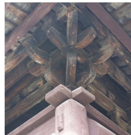
Figure 2.3f Corner Bracket Set of waiyan puzuo , Main Hall, Bao'ensi
