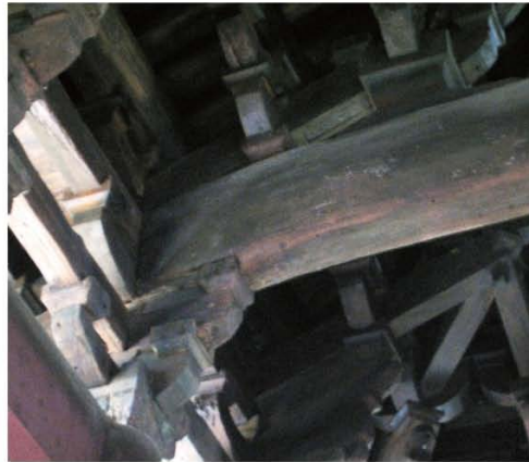
Figure 1.1h Picture of the rear view of capital set, Main Hall, Yanfusi
