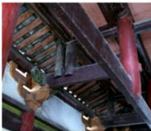
Figure 2.7n Two-rafter beam connecting the interior column to the eave column of the side, Pingxianglou
