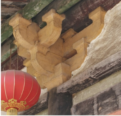
Figure 2.7e Picture of a capital set, Pingxianglou.
