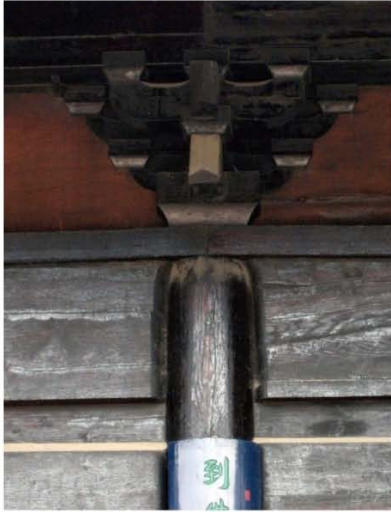
Figure 1.3e Picture of capital set on facade, Main Hall, Zhenrusi
