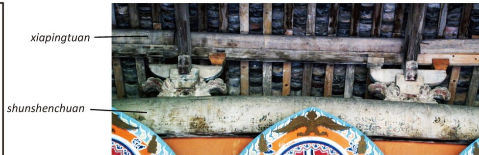
Figure 2.4h Bracket sets between Shunshenchuan and Xiapingtuan , Main Hall, Yong'ansi
