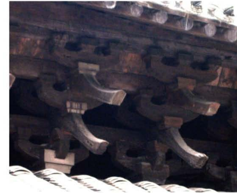
Figure 1.1i Picture of the front view of capital(right) and intercolumnar(left) sets, Main Hall, Yanfusi
