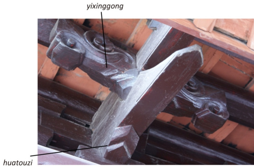
Figure 2.8d Bottom view of the intercolumnar set on the facade, Pantuoshidian, Qiqushan Damiao
