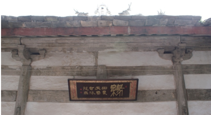
Figure 2.1c Bracket sets on the rear elevation, the Main Hall of Lifengguan
