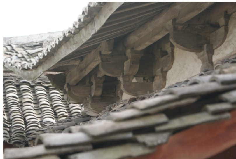
Figure 2.1d Bracket sets on the side elevation, the Main Hall of Lifengguan
