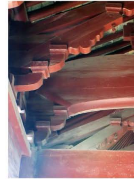
Figure 1.6e Rear view of capital set, Main Hall of Xuanyuangong
