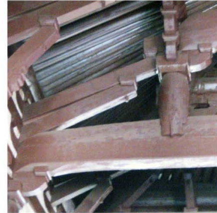
Figure 1.2h Rear view of capital set, Main Hall of Tianningsi
