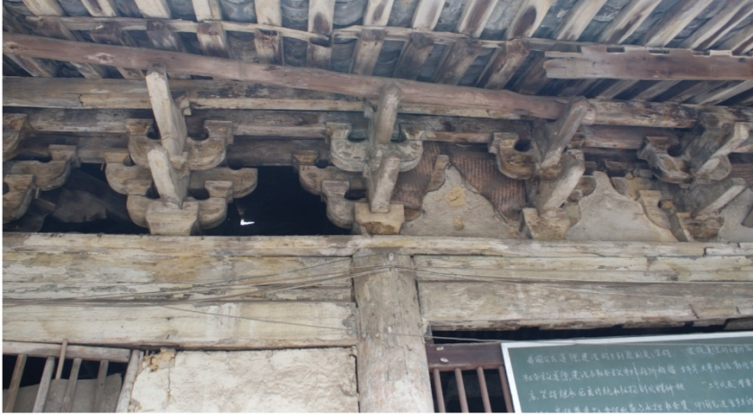
Figure 2.11d Picture of the capital set and the intercolumnar set on the facade, the Main Hall, Dubaisi
