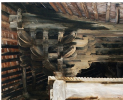
Figure 2.5d Corner set, Wenchangdian, Wulongmiao
