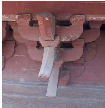
Figure 1.6f Front view of capital set, Main Hall of Xuanyuangong
