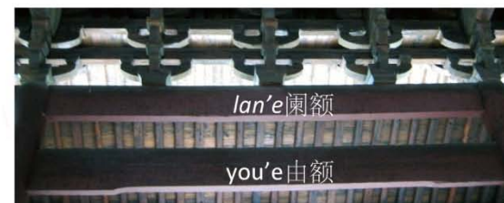
Figure 1.1n Picture of lan'e and you'e, Main Hall, Yanfusi
