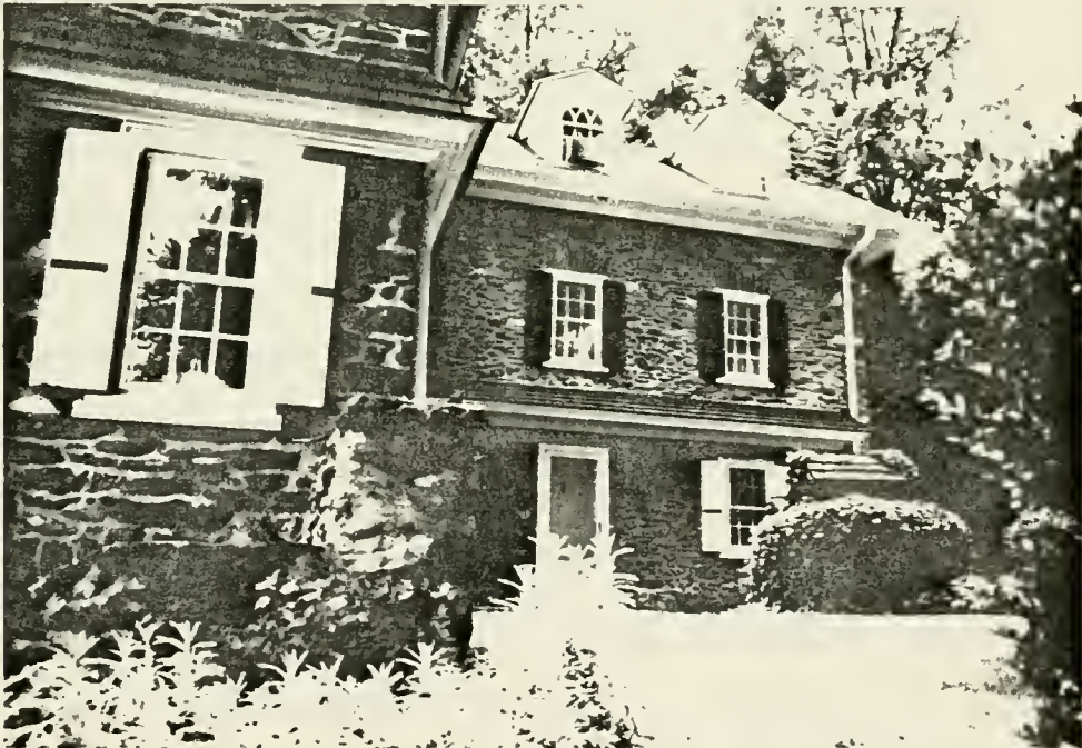
Figure 44: New Pent Eave on the north facade original/western section (note removal of portico shown in Figure 19) Photograph 1990.
