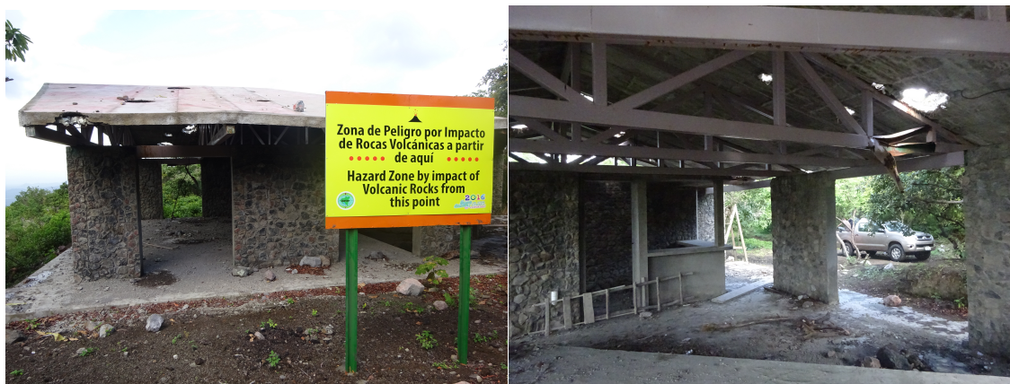
Figure 6 Image taken following the November 2015 volcanic eruption. The roof sustained significant damage, and its structural integrity was threatened (Bridges 2016).
