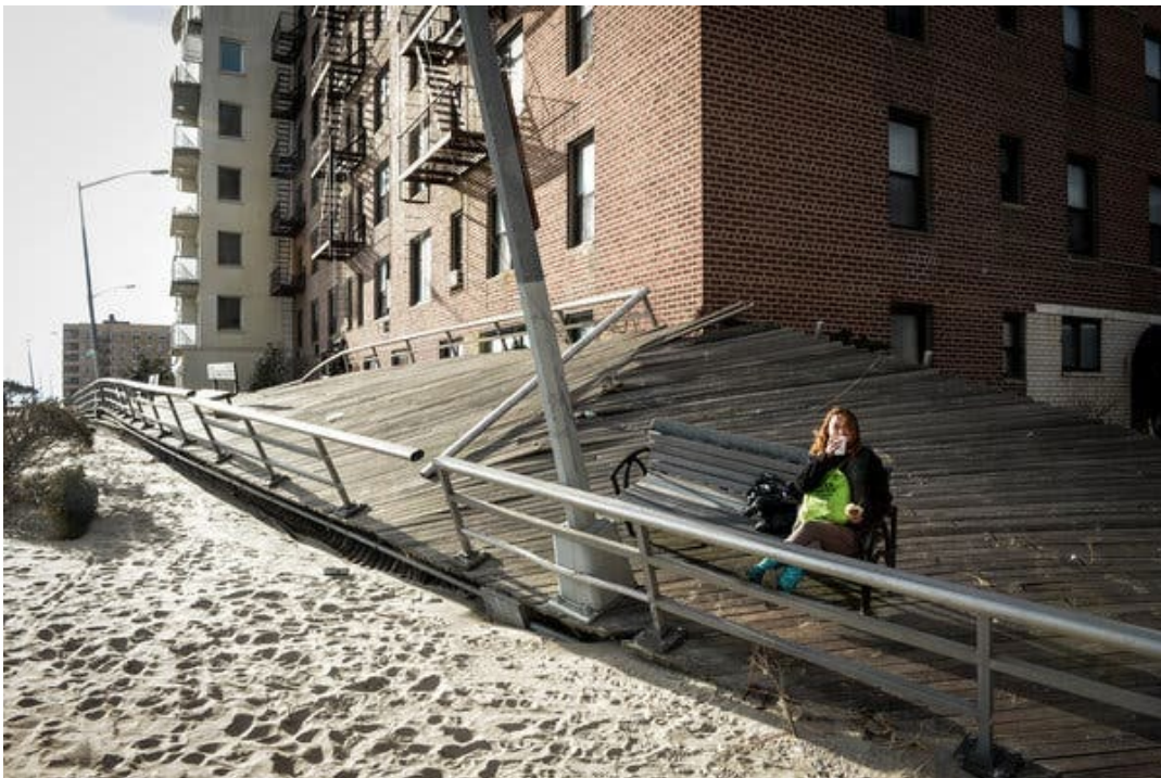
Figure 16, Rockaway Boardwalk damage after Hurricane Sandy, Source: The New York Times .
