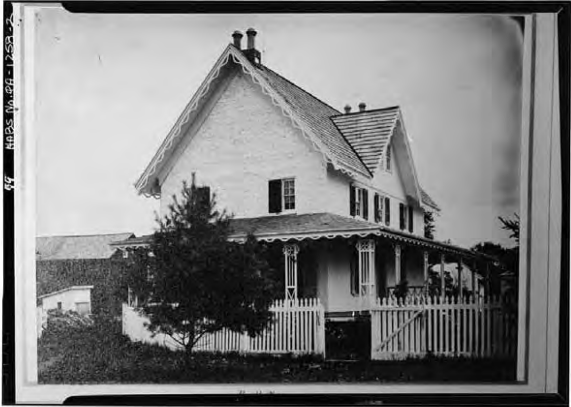
FIGURE 9 – The Brinton 1704 House, c.1870, with nineteenth century additions. (Image: Historic American Buildings Survey)
