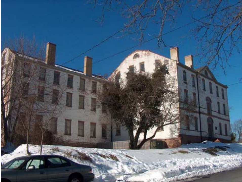
Figure 2. South wing of Proprietary House, 2005
