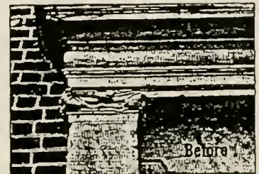
Pohick Church, Ft. Belvoir, V.A. Cast replacement capitals using Jahn M150 - special dry casting mortar
