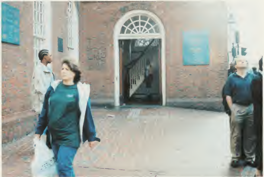
Figure 5 - Old South Meeting House, Boston, MA. The area in front of the door has been re-graded to allow wheelchair access. Other doors retain the historic steps.
