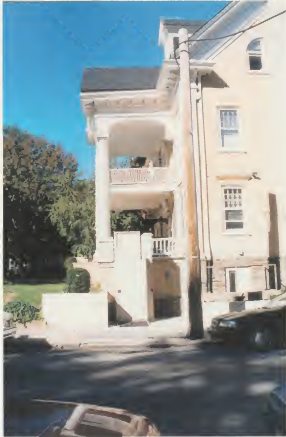
Figure 9 - 4601 Spruce Street, Philadelphia, PA. This wheelchair lift provides access onto a porch that is five steps above grade. It is shielded from view by a low wall and landscaping.
