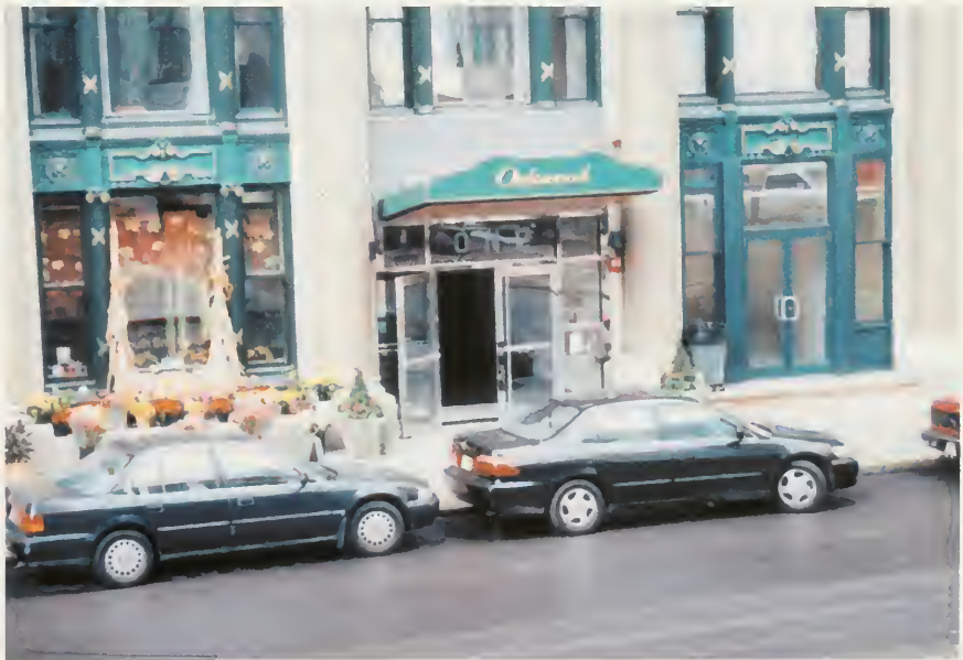
Figure 7 - The Oakwood, Boston, MA. The original front door has been lowered to grade level. The area above has been in-filled with corrugated metal.
