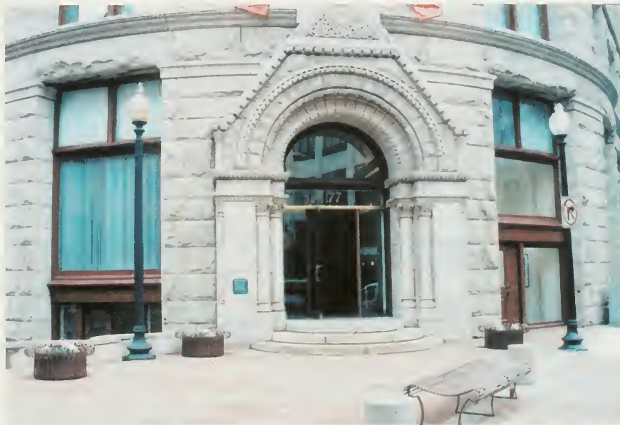
Figure 6 - The Beal Building, Boston, MA. The window on the right of the entrance has been replaced with a new accessible door which leads to an elevator lobby.
