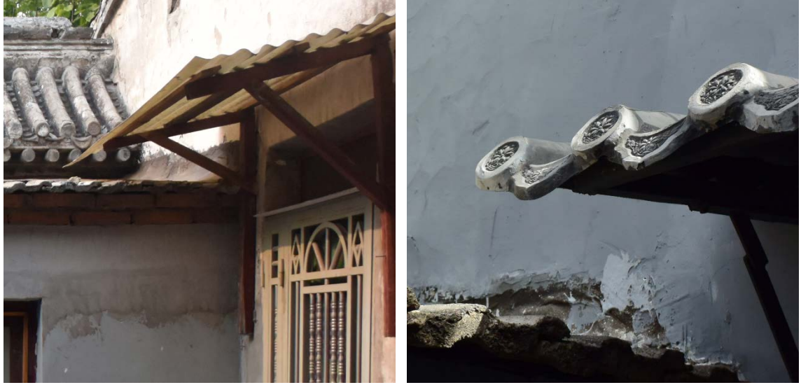
Figure 37. Roof-tiles. Before : Large pan tiles and plastic canopy, used for a makeshift addition at the entrance of a courtyard (left); After : Small antique pan tiles, renovated by SHHPS (right). Photo by Haoyu Wang, Beijing, July 2015 (left) and March 2016 (right).
