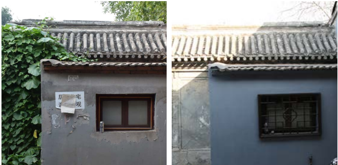
Figure 38. Window sash. Before : No stylistic details on the addition in front of the screen wall (left); After : A newly installed hollow window sash for the re-painted structure (right). Photo by Haoyu Wang, Beijing, July 2015 (left) and March 2016 (right).
