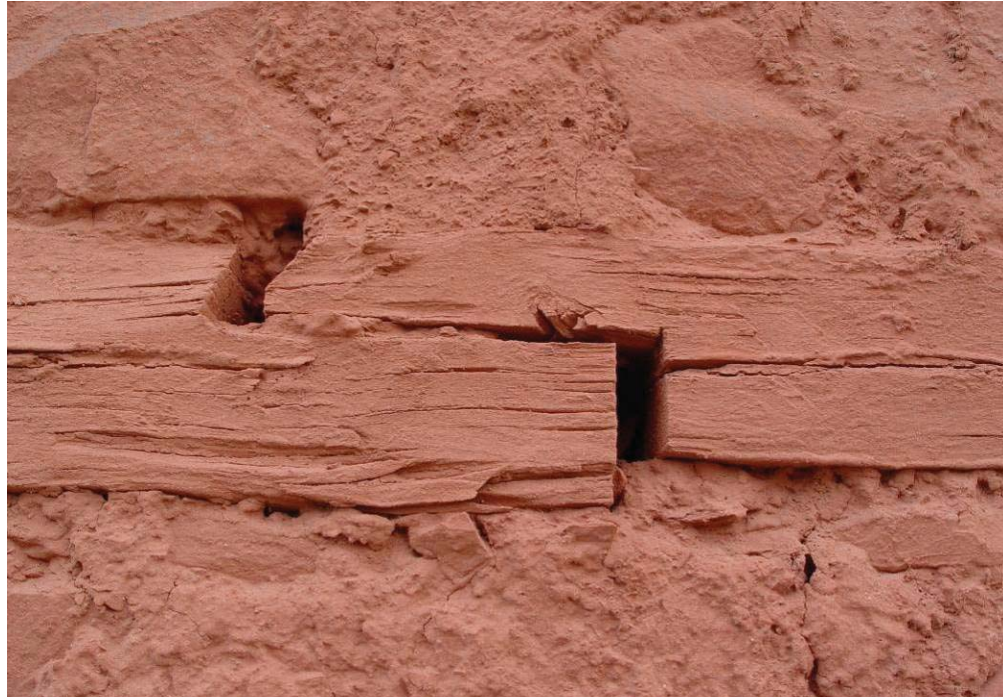
Figure 7 Joint detail - Wooden ring beam, Themisgam, Ladakh
