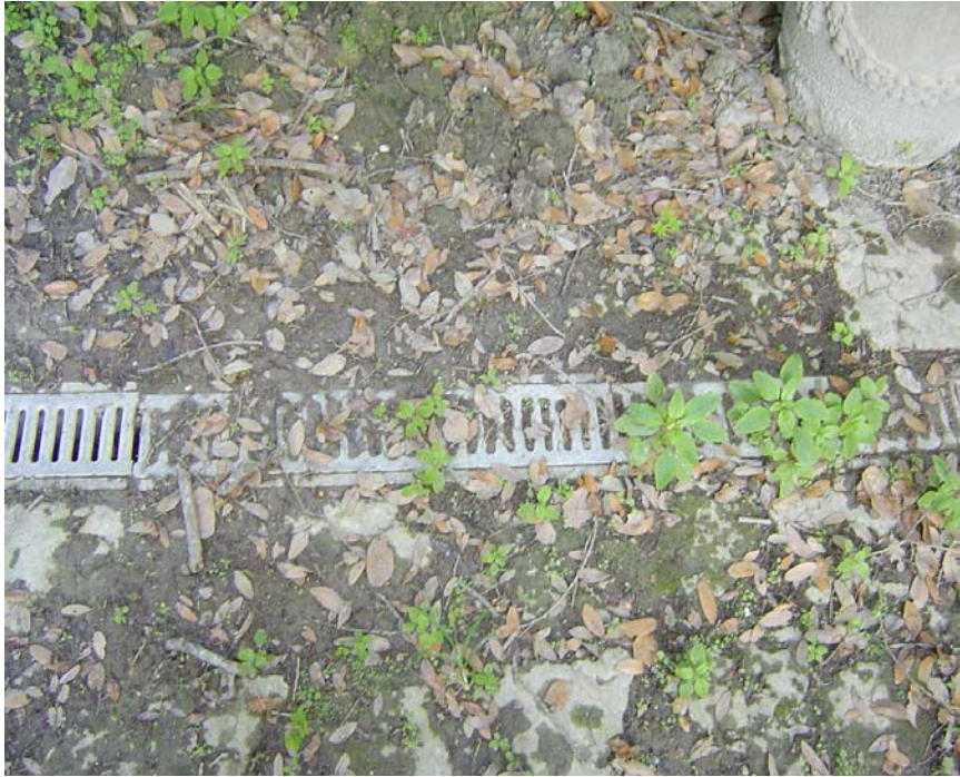
Fig.33 Clogged drains in the Marine garden, (summer 2003)
