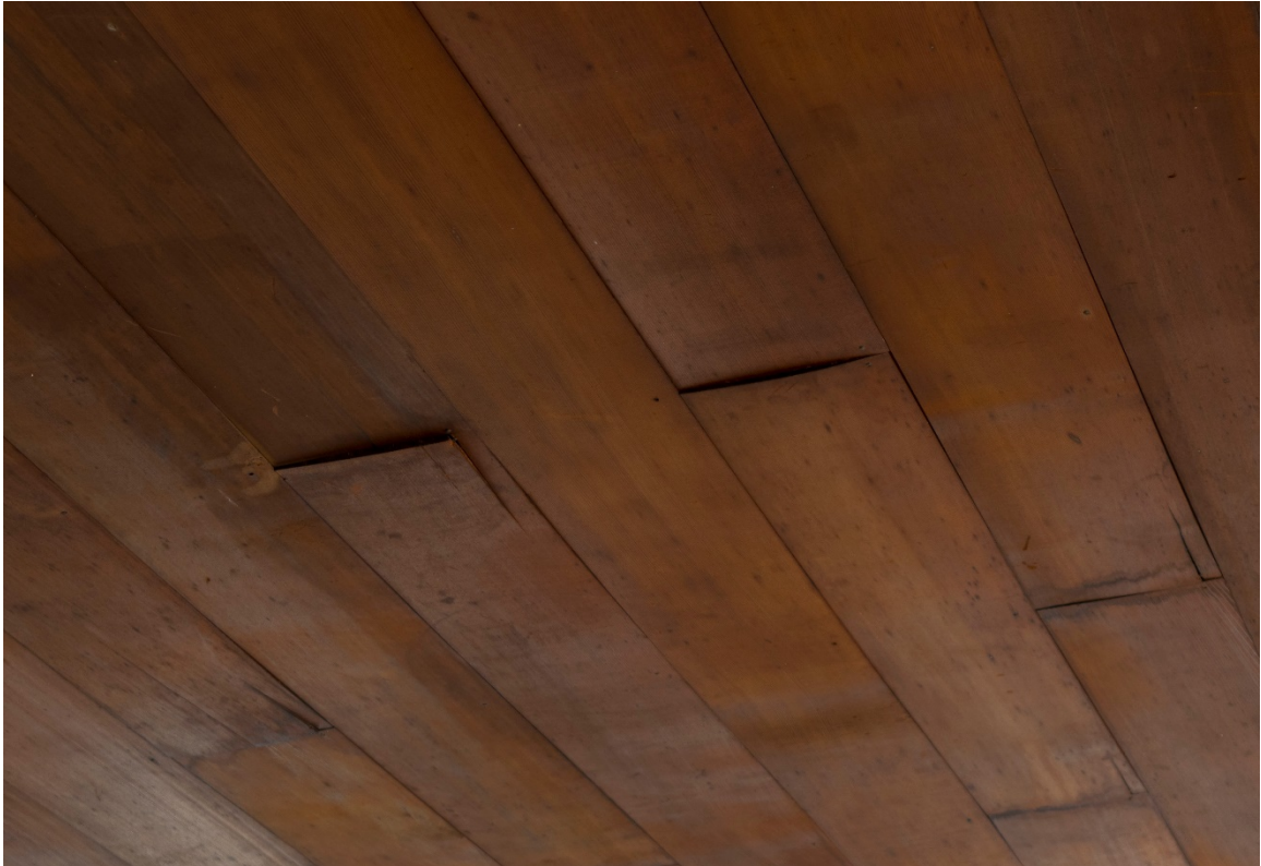
Figure 38. Example of cupping cedar boards after water infiltration, creating a larger opening. Source: Author, January 26, 2018.
