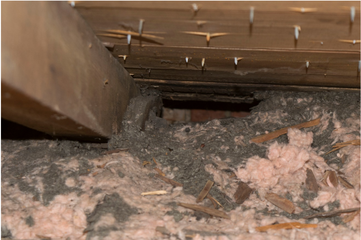
Figure 37. Image taken in the attic space showing holes between the roof decking and the cedar ceiling. Hole has presence of dirt and black staining on the wood, indicating the presence of water. Source: Author, April 10, 2018.
