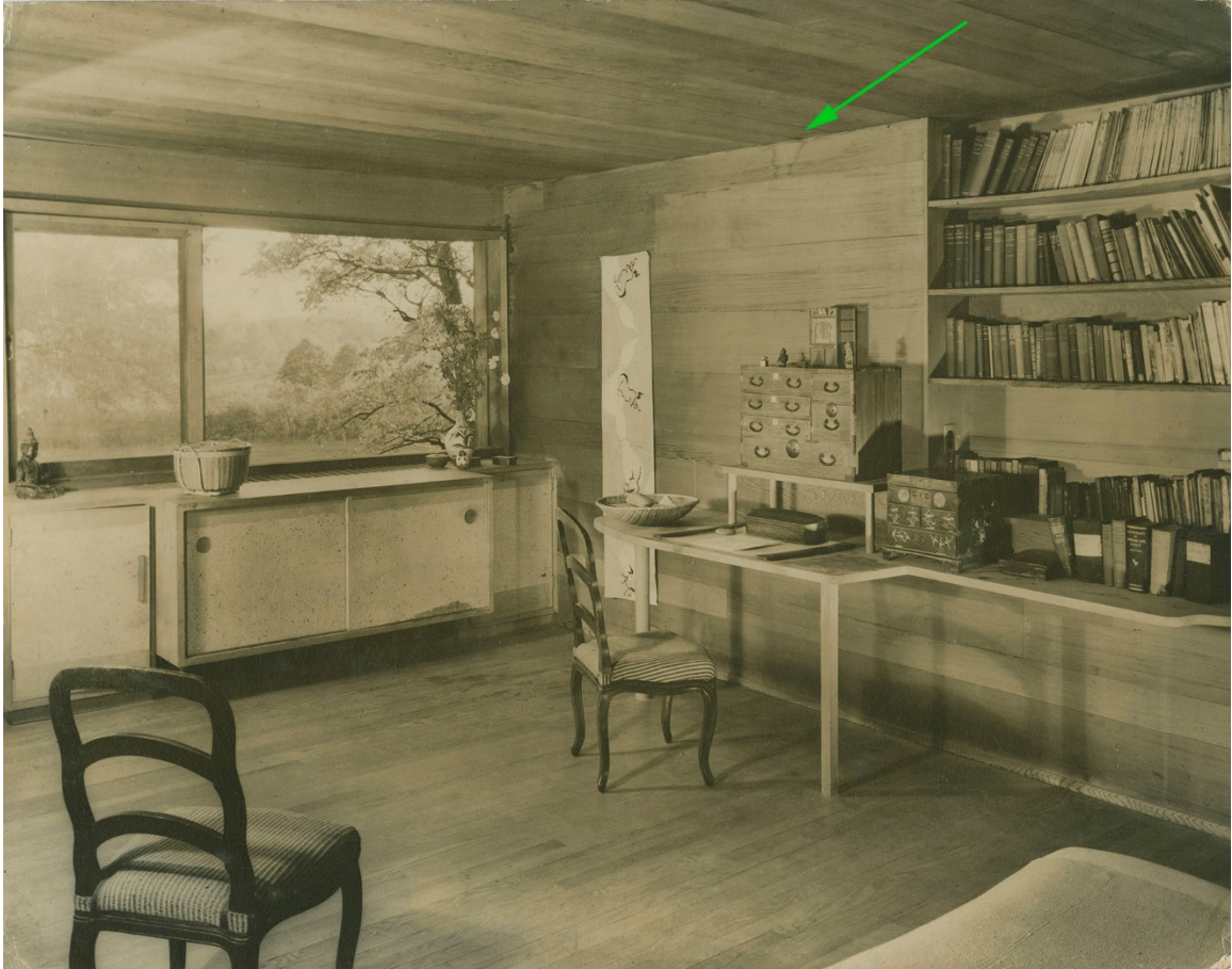
Figure 31. Photograph of a water stain on the cedar interior, indicated by a green arrow. Source: Raymond Collection, University of Pennsylvania Architectural Archives, indicator arrow added by author.
