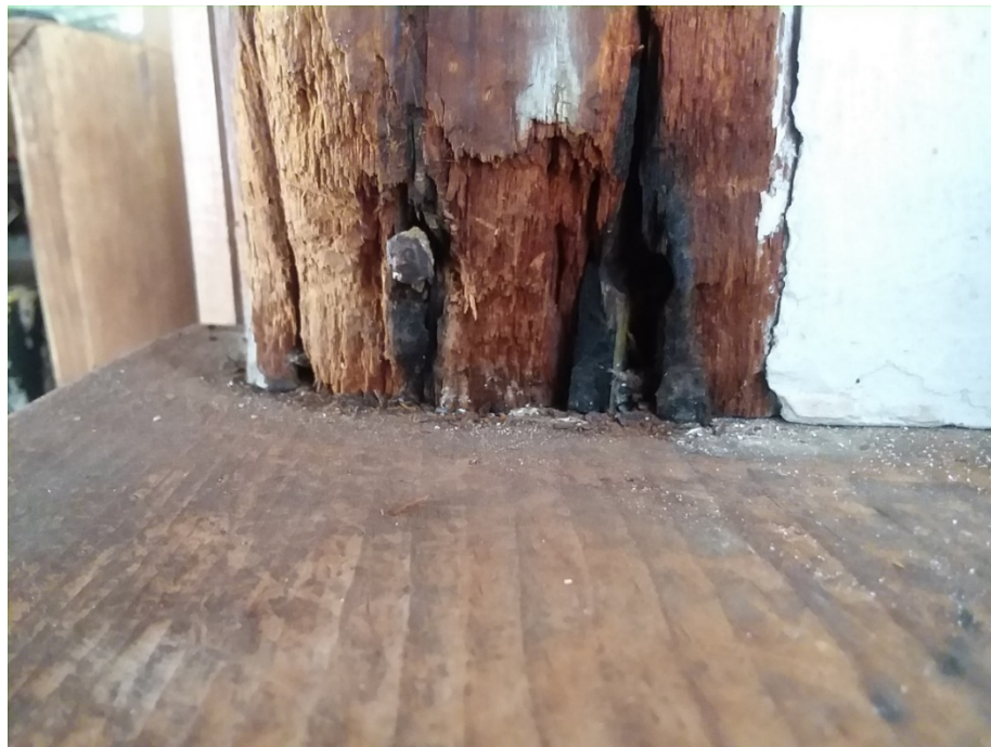
Figure 36. Black staining on a wood window surround due to untreated iron in wrought nails. Source: Author, March 27, 2018.
