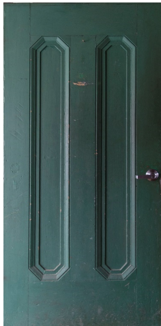
Figure 29. Style of door used on the first-floor main openings on the north and south elevations. Distinctive elongated hexagonal moulding is applied to the panel with small finishing nails, inferring they were constructed in the early-mid 1800s. Source: Author.
