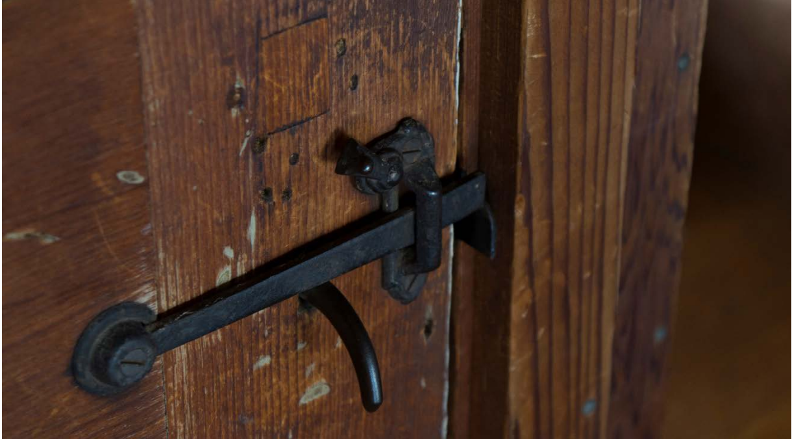
Figure 25. Cast iron thumb latch located on a third-floor hallway closet. The downturned lift indicates it was produced after 1800. The handle is on the interior, indicating the door was moved to its current position in the Raymond campaign. Source: Author, March 16, 2018.
