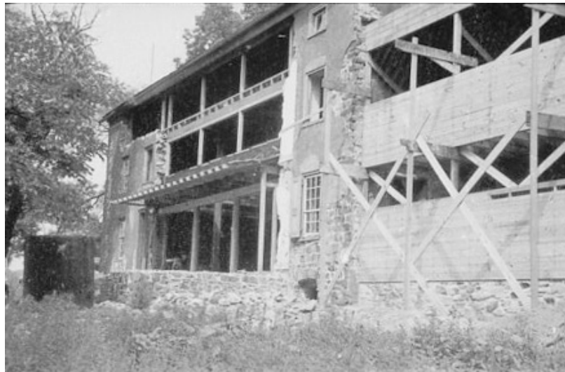
Figure 13. Construction photograph of the south elevation showing areas of the masonry envelope that were removed, and the new wood addition on the east façade. Source: Sugiyama Collection, University of Pennsylvania Architectural Archives.
