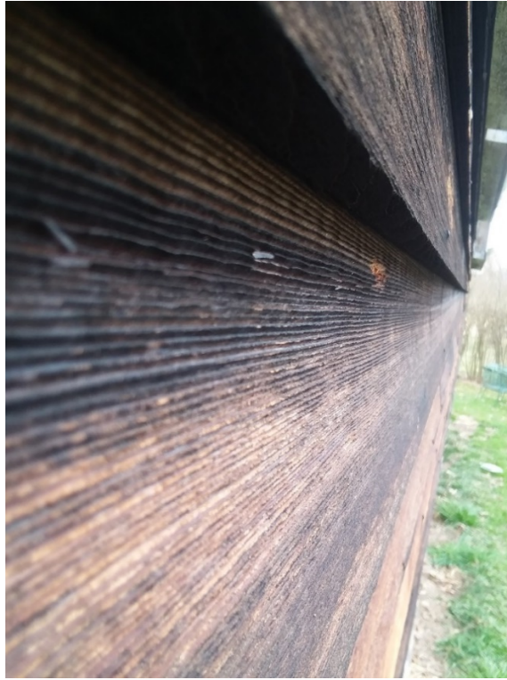
Figure 33. Raking view of decayed earlywood and therefore raised latewood in exterior cedar shiplap due to UV damage. Source: Author, March 27, 2018.
