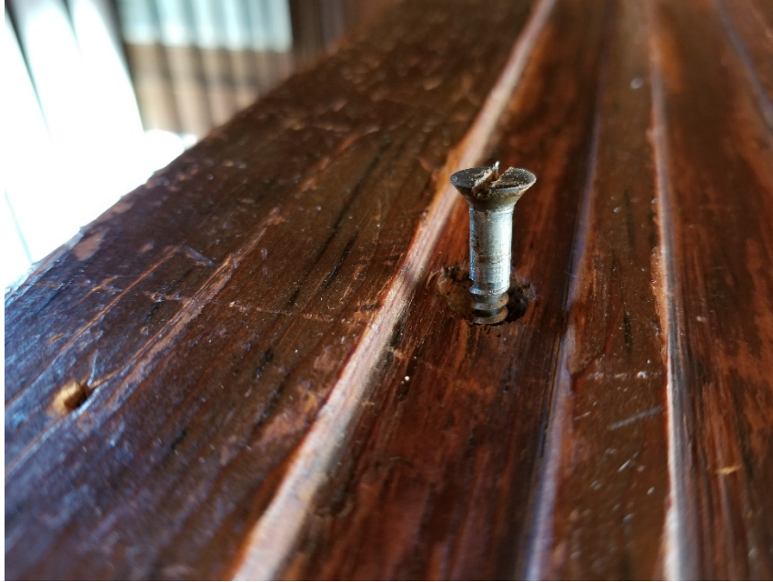
Figure 22. Screw extracted from the mezzanine-level fusuma track that creates the division between the hallway and lightwell area. Source: Author.
