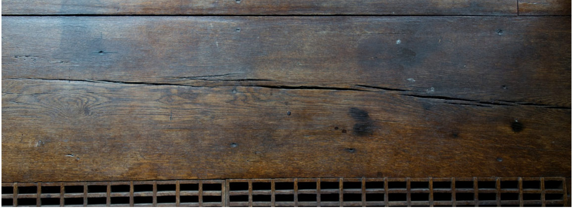
Figure 35. Floor board near the center of the panel of glass doors on the first floor shows increased rate of checking compared to other boards due to cyclic exposure to sunlight.
