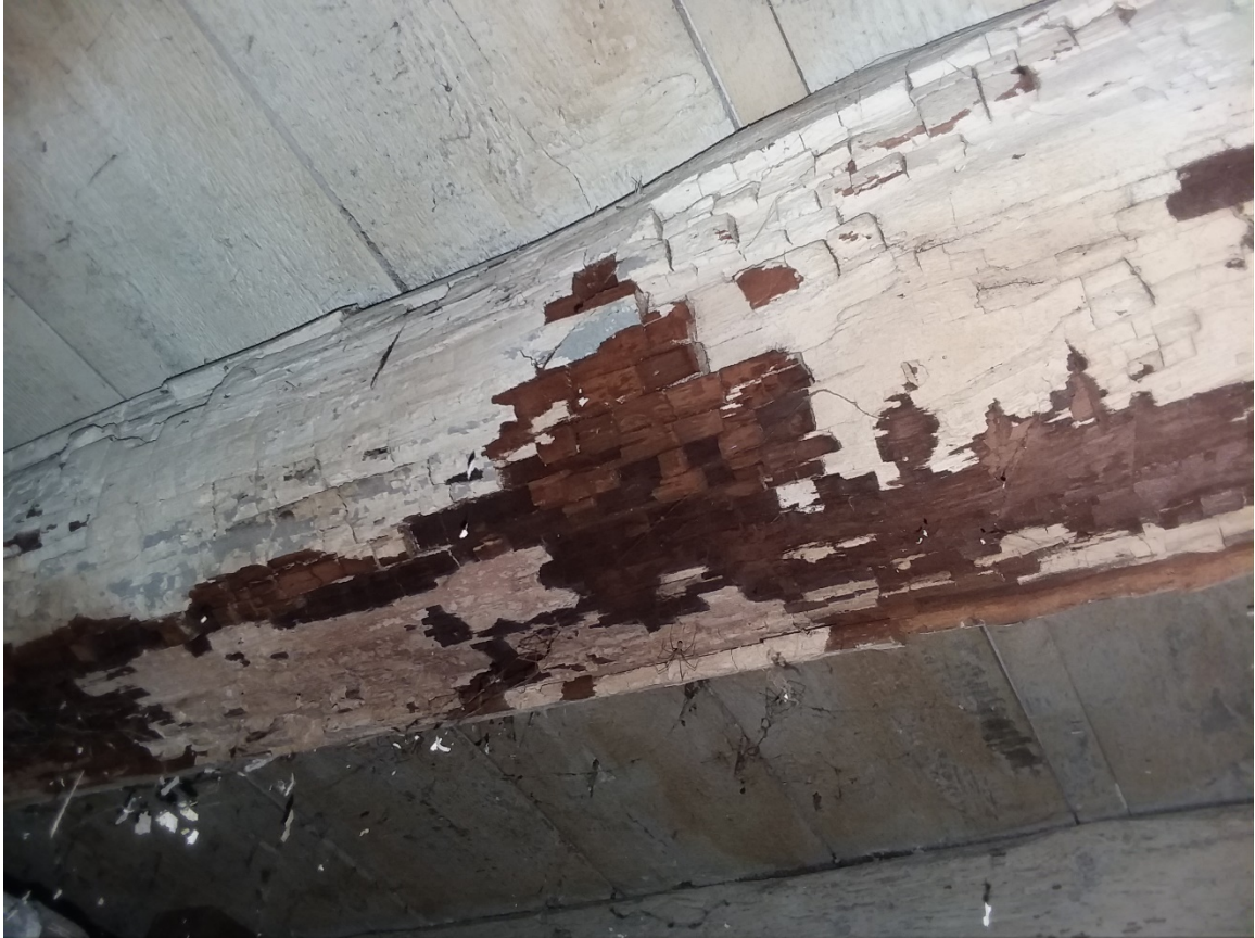
Figure 34. Basement joist showing classic checkerboard pattern indicative of a type of brown rot. Source: Author, March 27, 2018.
