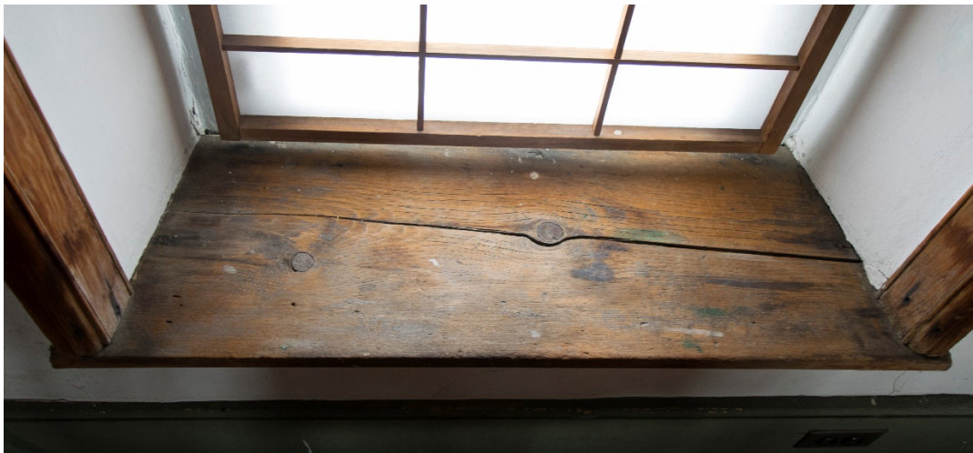
Figure 32. Showing checking of the wood sill and loss of color due to UV light. Source: Author, April 10, 2018.
