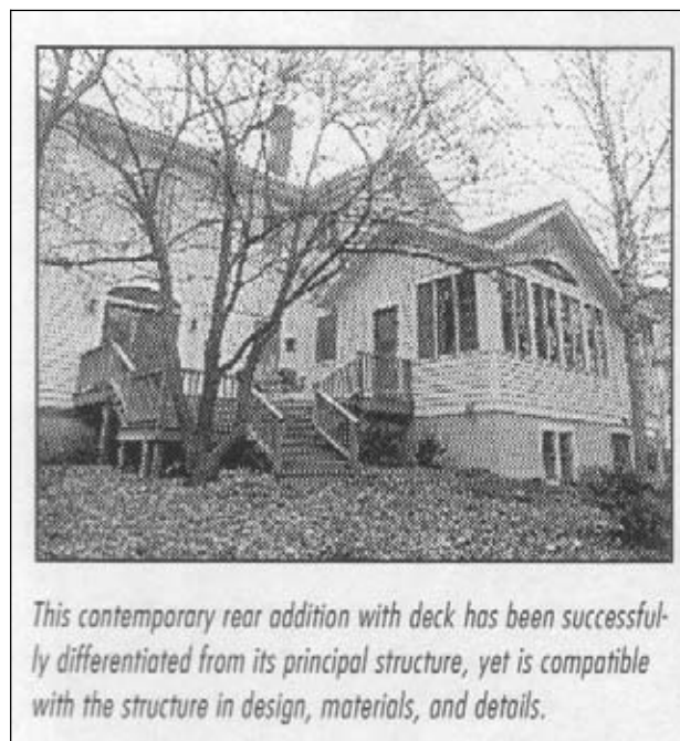
Figure 7 – The problematic form of the deck as well as the design of the addition make this a questionable example of an appropriate addition in the Design Guidelines for Raleigh Historic Districts . 39
