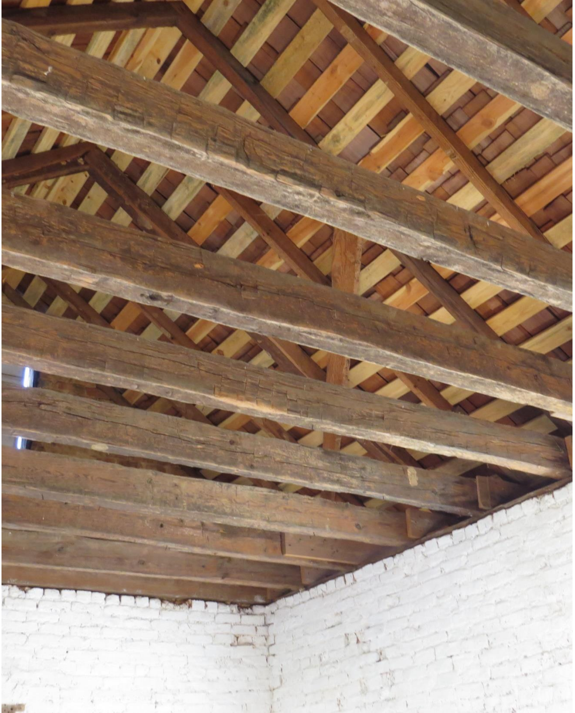
Fig. 1.17: View of both the 19 th century and replacement framing members of the roof structure of the original slave dwelling. (Harper, 2019)
