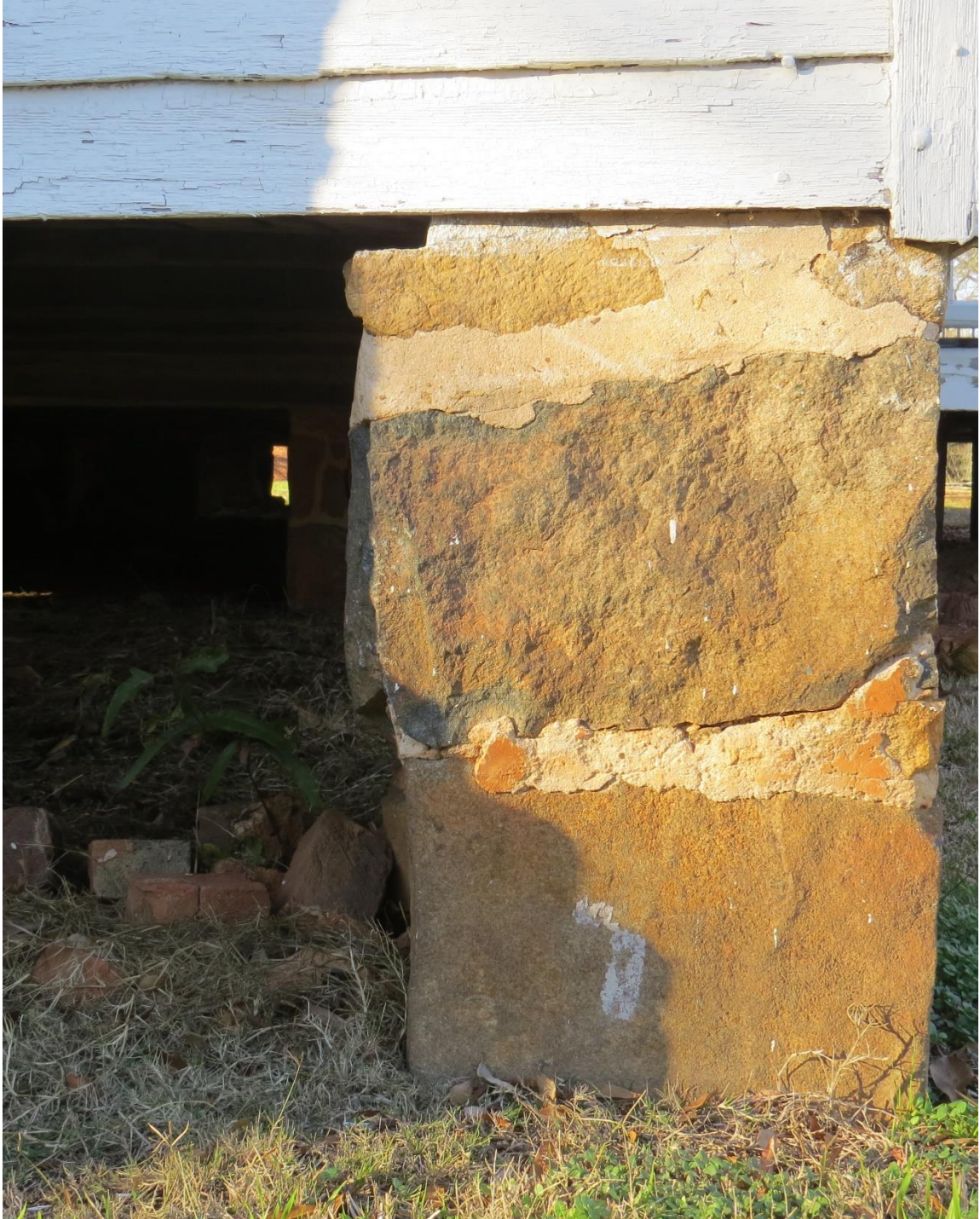
Fig. 1.3: Stone “piedmont piers” beneath the Homestead House. (Harper, 2019)
