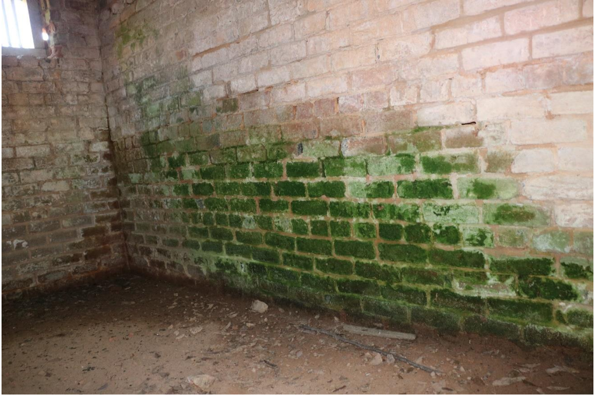
Fig. 1.25: View of biomaterial above the leftmost arch in the northern wall of the cellar. (Photograph taken by Sara Johnson of Historic Brattonsville)
