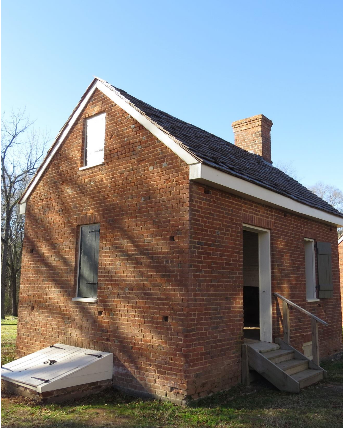
Fig. 1.10: Perspective view of the original dairy alluding to the structure's multiple uses. The reconstructed bulkhead doors (bottom left) lead to the cellar for milk cooling and storage, the main floor was likely used as both a living space and work room, and the window opening within the gable end allows for light to enter the loft. (Harper, 2019)
