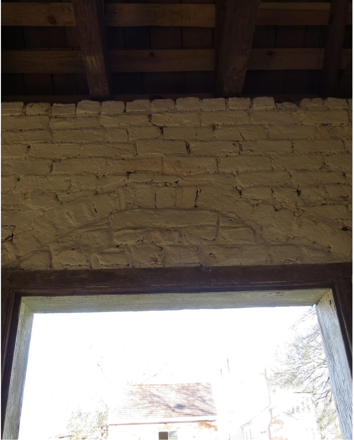
Fig. 1.14: View of the jack arch spanning the doorway of the original slave dwelling. (Harper, 2019)
