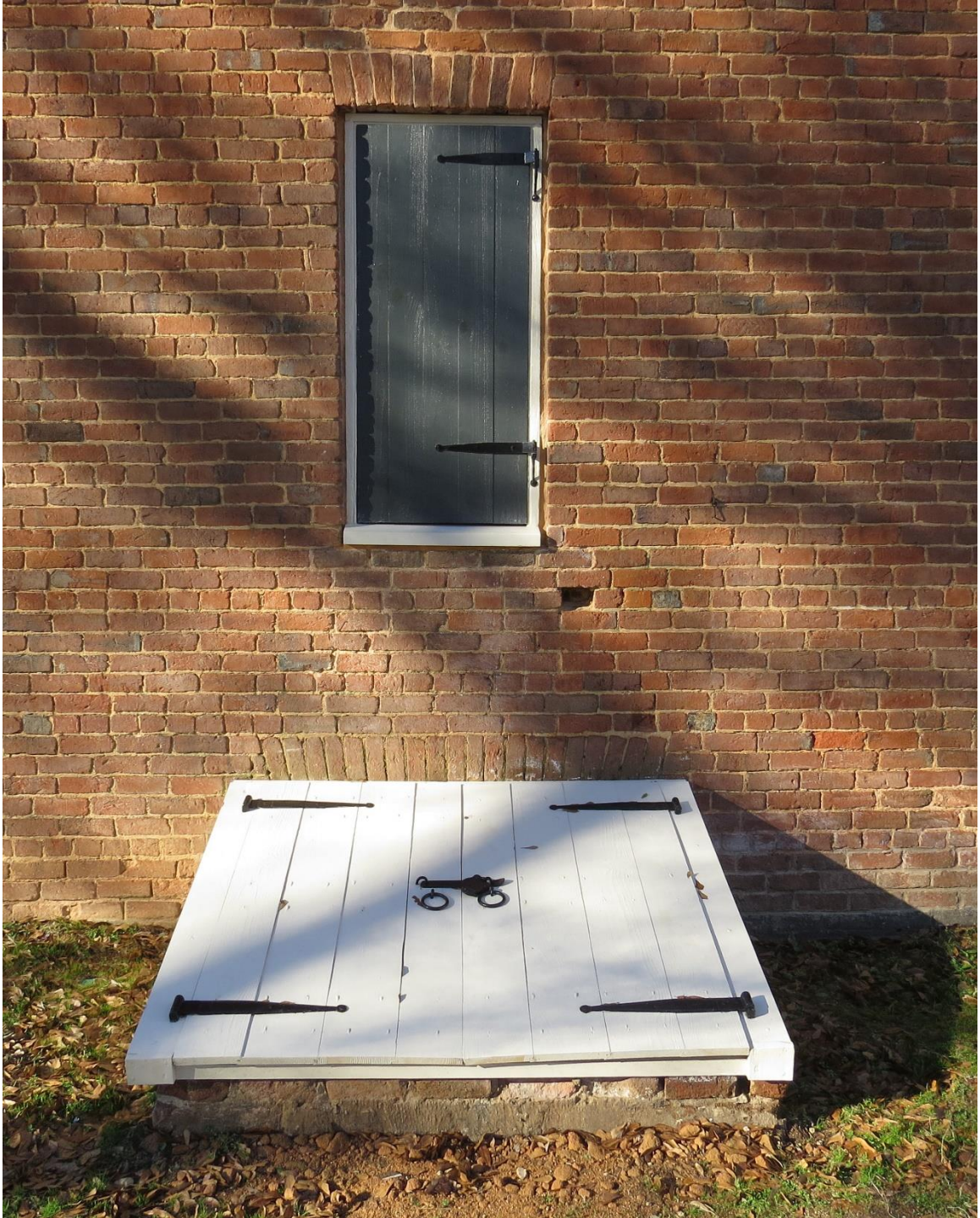
Fig. 1.21: View of the reconstructed bulkhead doors leading to the cellar of the original dairy. (Photograph taken by Sara Johnson of Historic Brattonsville)
