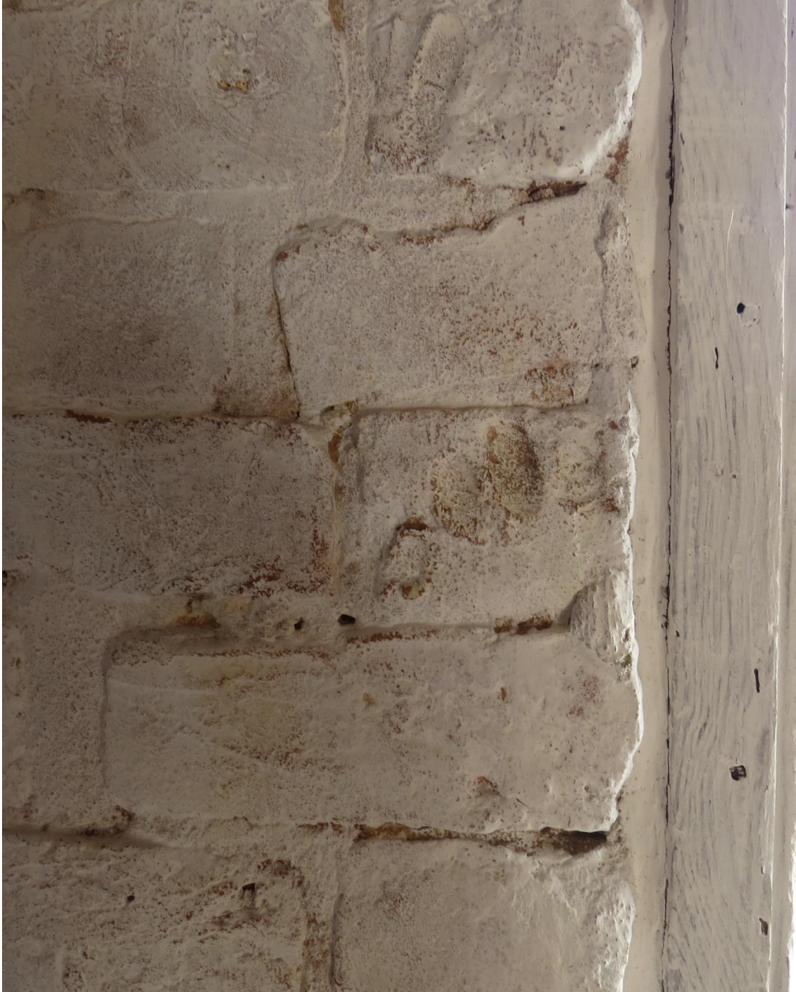
Fig. 1.27: Fingerprints in the original dwelling left by the slaves who pressed the clay into the brick mold. Seen at the center and top of the image. (Harper, 2019)
