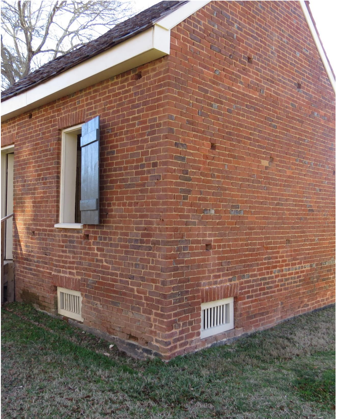
Fig. 1.11: Perspective view of the original dairy emphasizing two of the three grilled vents at the base of the structure. (Harper, 2019)
