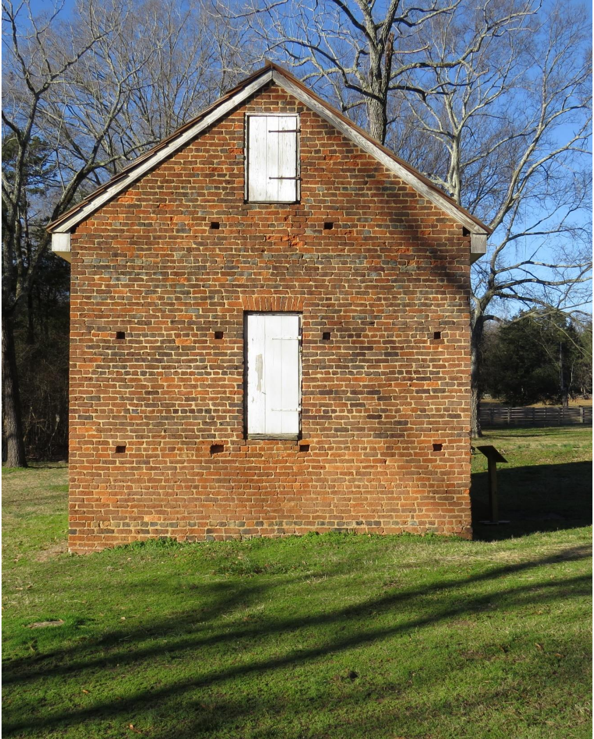
Fig. 1.15: View of the eastern wall of the original slave dwelling with visible putlog holes. (Harper, 2019)
