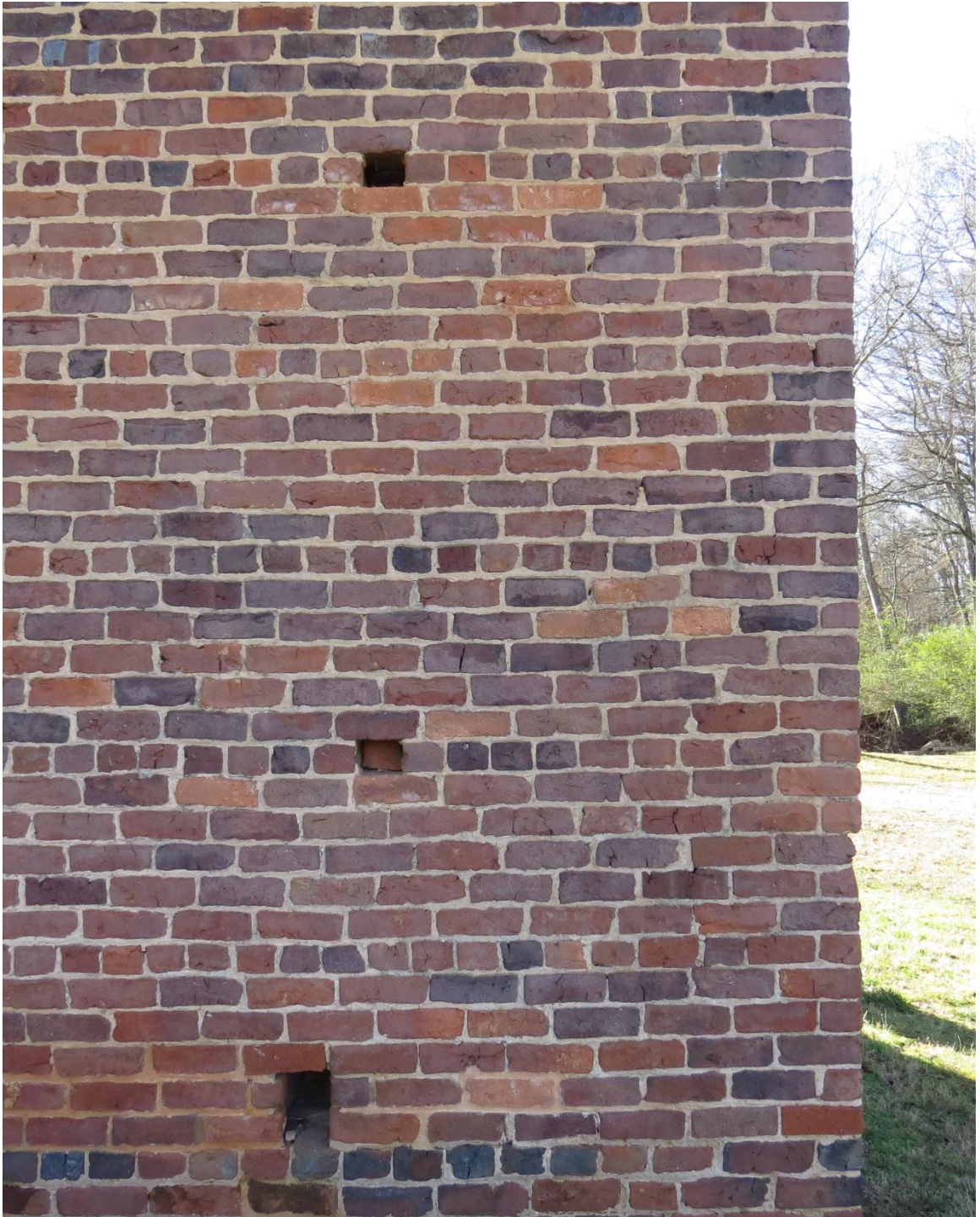
Fig. 1.16: Putlog holes in the northern wall of the original dairy. (Harper, 2019)
