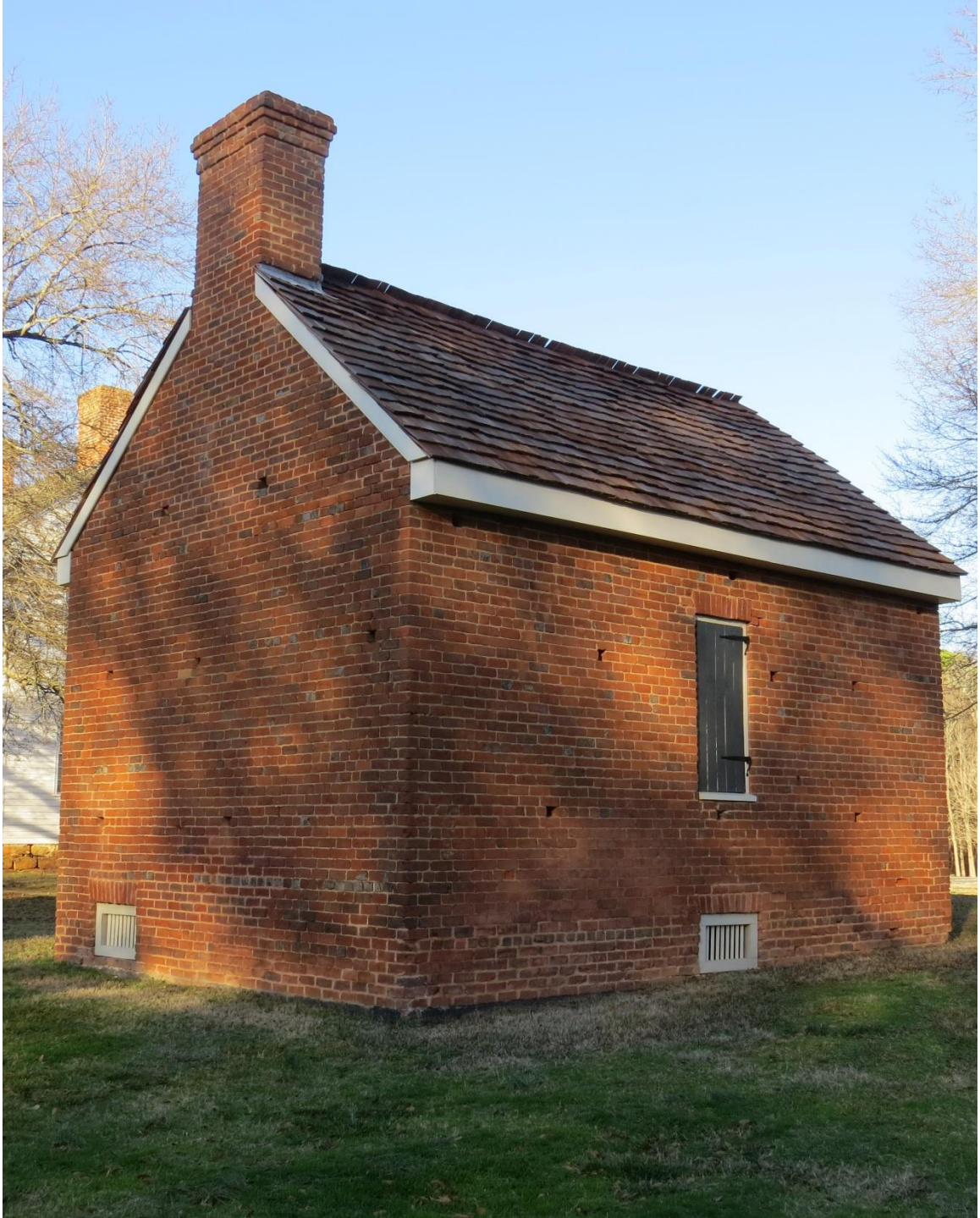
Fig. 1.20: Perspective view of the original dairy illustrating the grilled vents in the base of the southern and western walls. (Harper, 2019)
