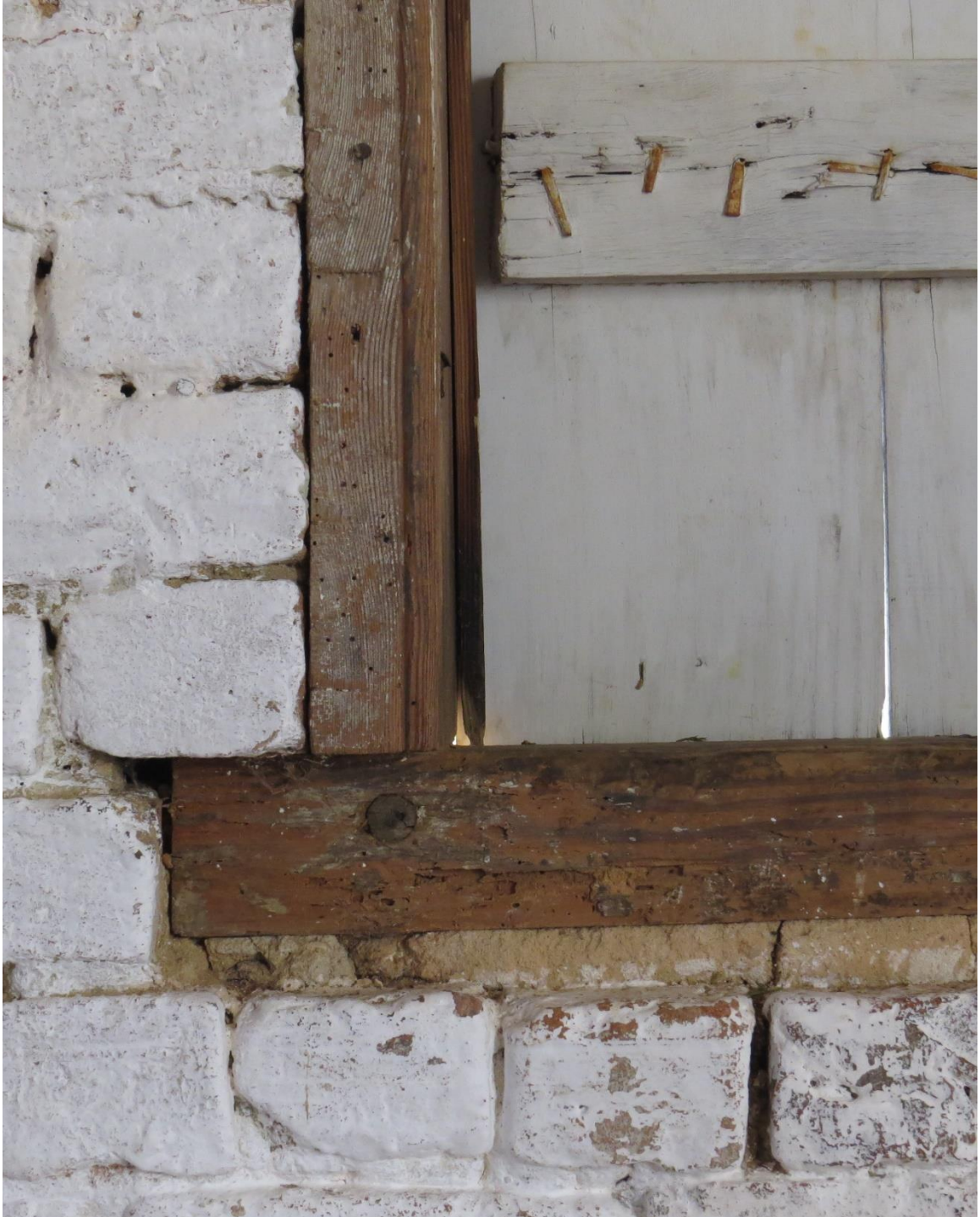
Fig. 1.26: View of the mortise and tenon joint of one of three original window frames in the original slave dwelling illustrating the craftsmanship of the slaves who lived within the domestic quarter. (Harper, 2019)
