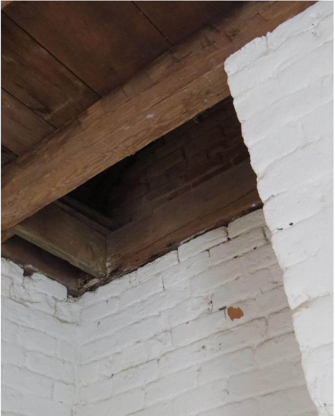
Fig. 1.18: View of the opening in the ceiling of the dairy's main room leading to the loft above. (Harper, 2019)
